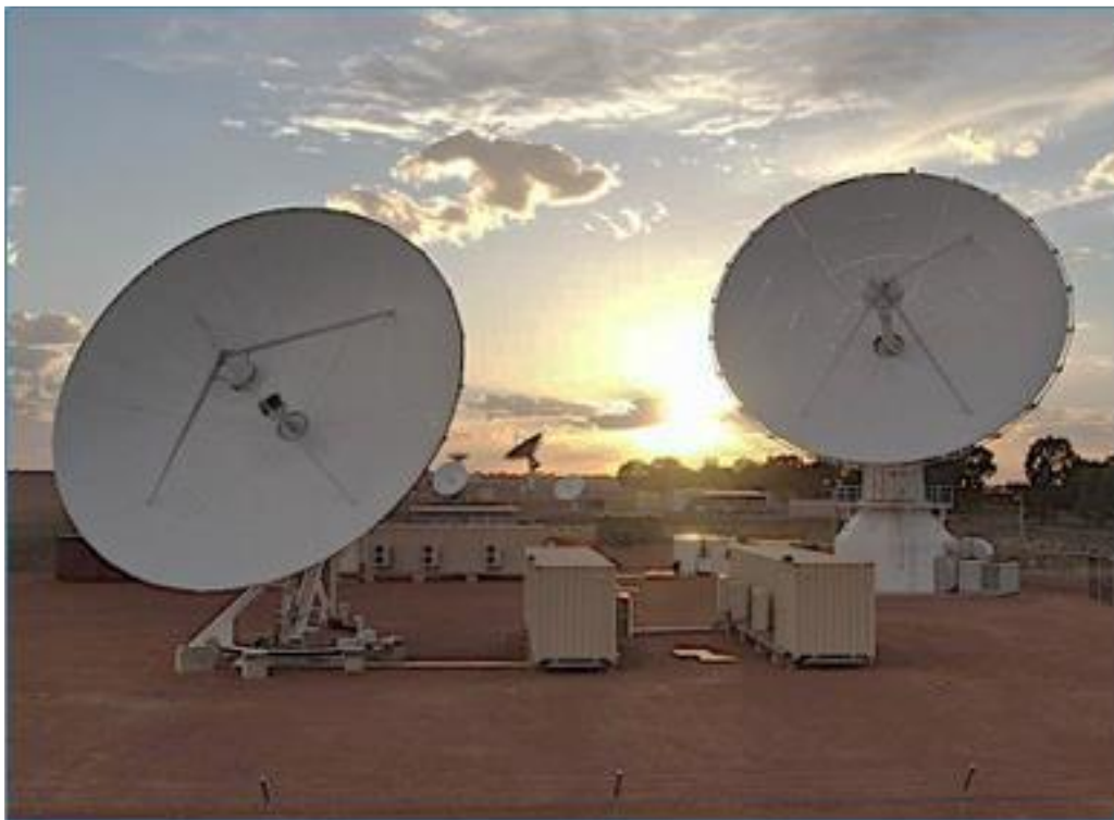
Figure 1. 16 m. and 13 m. diameter antennas for control and data downlink from U.S. Space Force EO/IR Weather System – Geostationary (EWS-G2) satellite, Dongara, Western Australia
