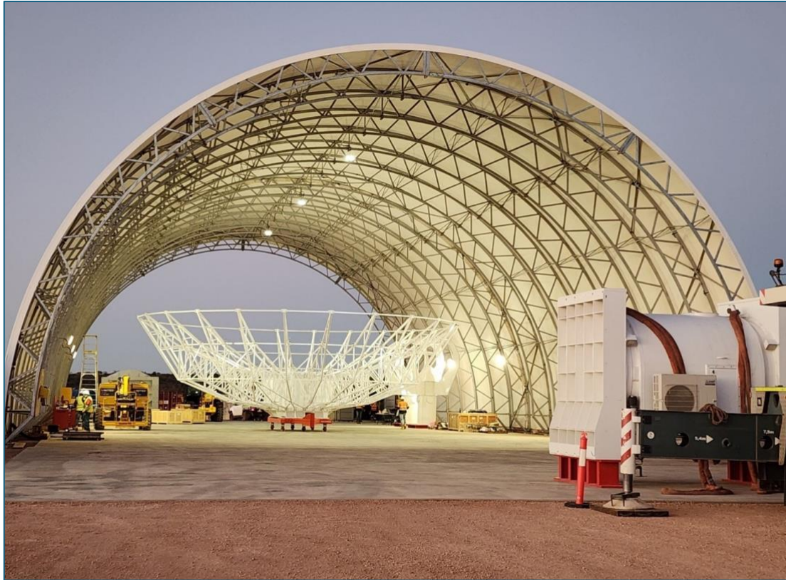
Figure 7. Deep Space Advanced Radar Site 1, Exmouth: one of 27 transmit and receive antennas under construction at the Antenna Integration Structure.
