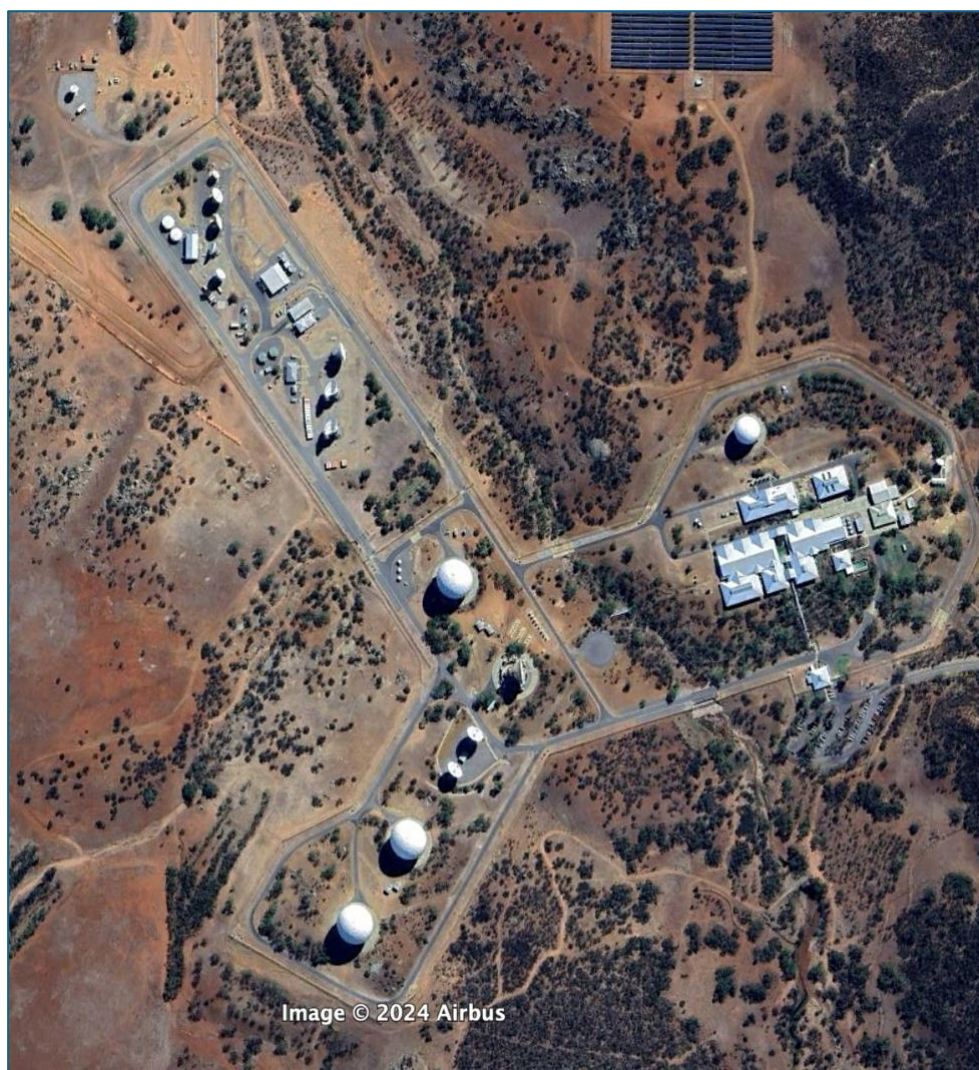
Figure 9. Australian Defence Satellite Communications Station, Kojarena, April 2024
