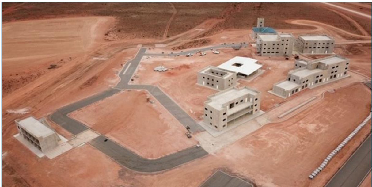
Figure 17. Urban Operations Training Facility, Cultana Training Area
