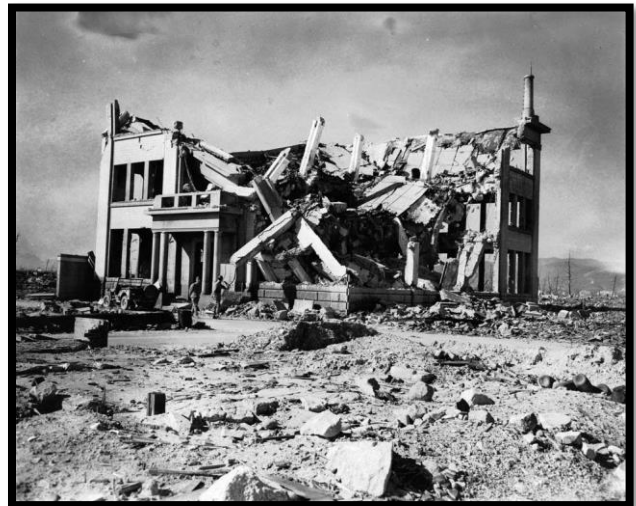
Figure 4-6: Impacts of Nuclear Blast on Wood-Framed House at Nevada Nuclear Weapons Test Site (5 psi) and on a Concrete Building at Hiroshima.
