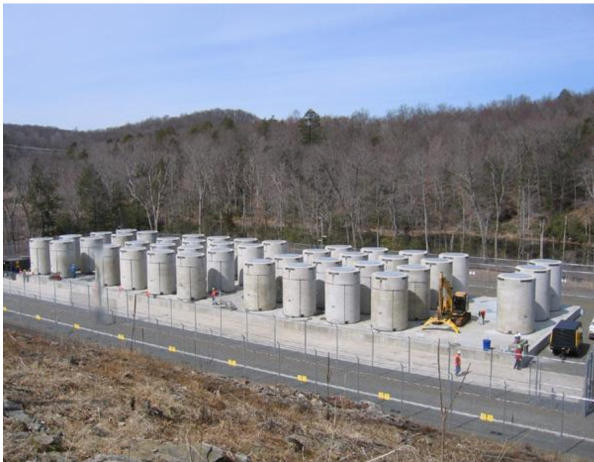
Figure 2-3: Dry Casks on a Concrete Pad at a US Reactor (Connecticut Yankee) 14
