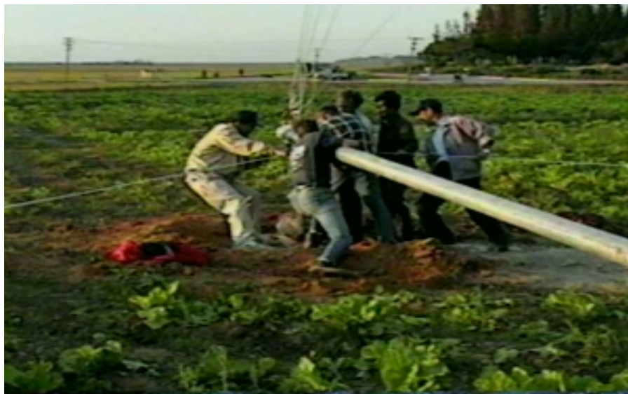
Hauling on the wind turbine tower.
