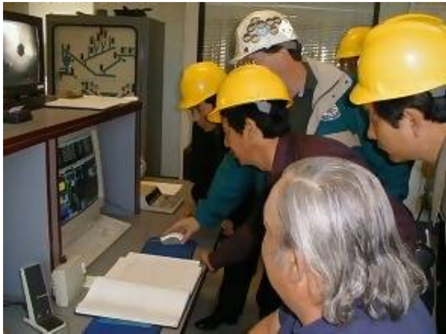
Inspecting monitoring equipment at Tracy Biomass Plant
