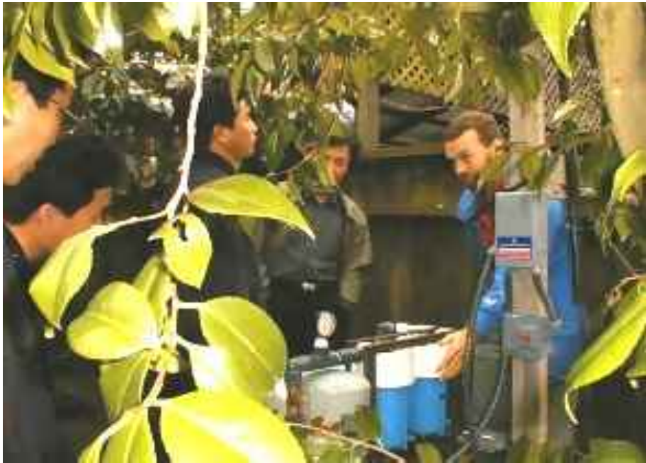
Inspecting installed ultraviolet water purification unit
