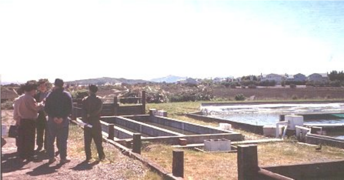
Visit to an Advanced Integrated Wastewater Ponding System at UC Berkeley Richmond Field Station.
