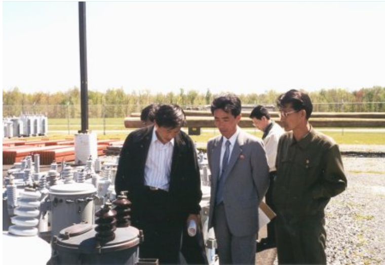
DPRK Delegation members inspect transformers at the Delaware Electric Cooperative in Greenwood, DE.
