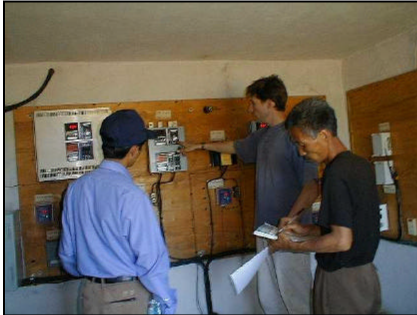
Figure 6: Training at Every Step, Every Level: Wind Turbine Power-house Training
