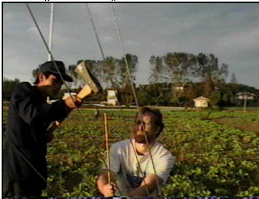
Figure 7: Installing "Ground Rods" at Unhari
