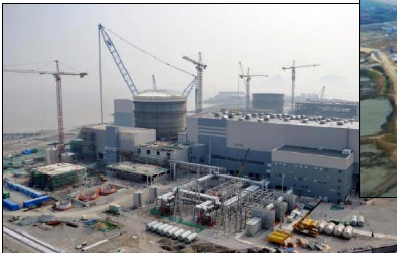
AP 1000 in Sanmen site (Sep. 2012)
