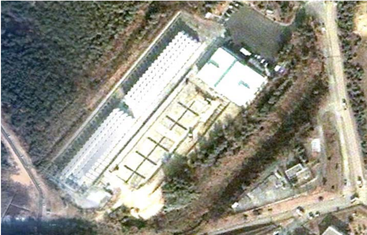
Figure 8. Concrete silo and MACSTOR/KN-400 at Wolsong (Google Earth, October 10, 2010)
