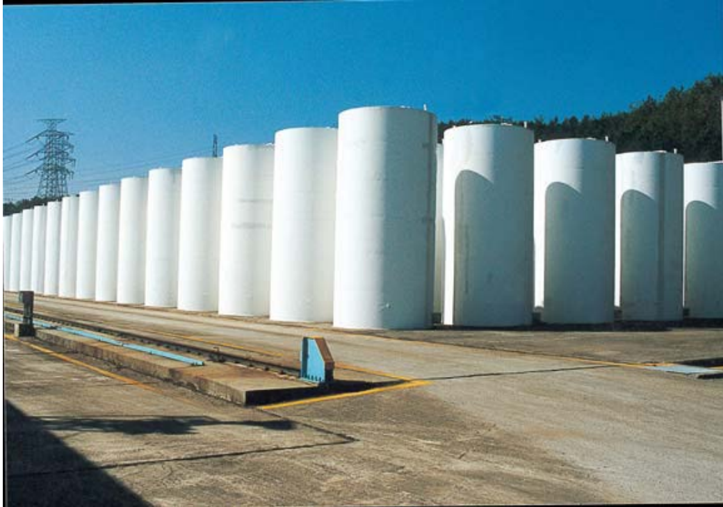
Figure 9. Concrete silo at Wolsong 15
