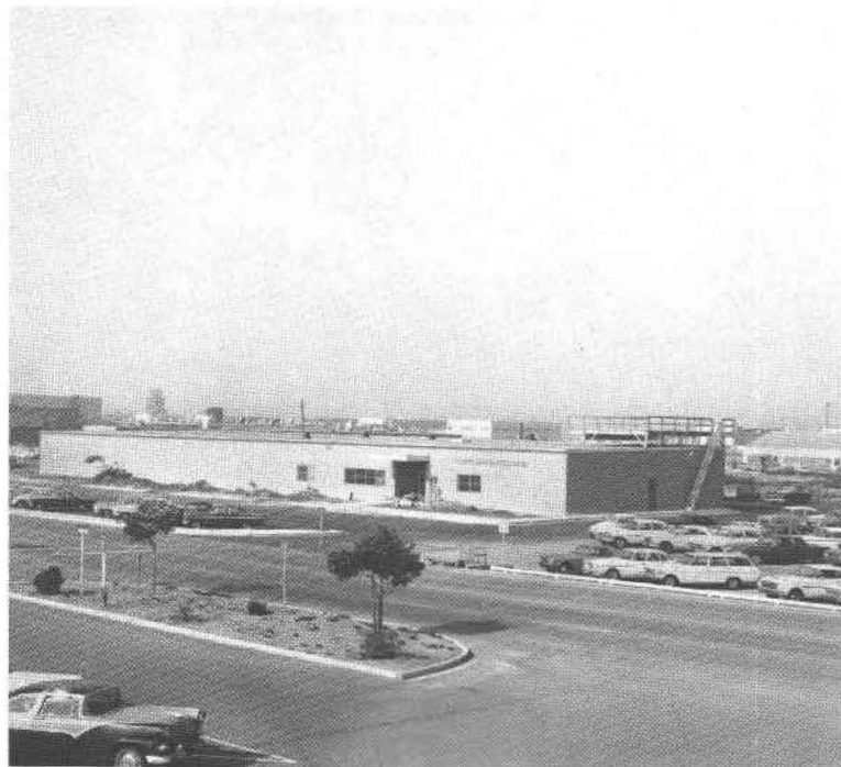
NAG Building during final phase of construction (1966).
