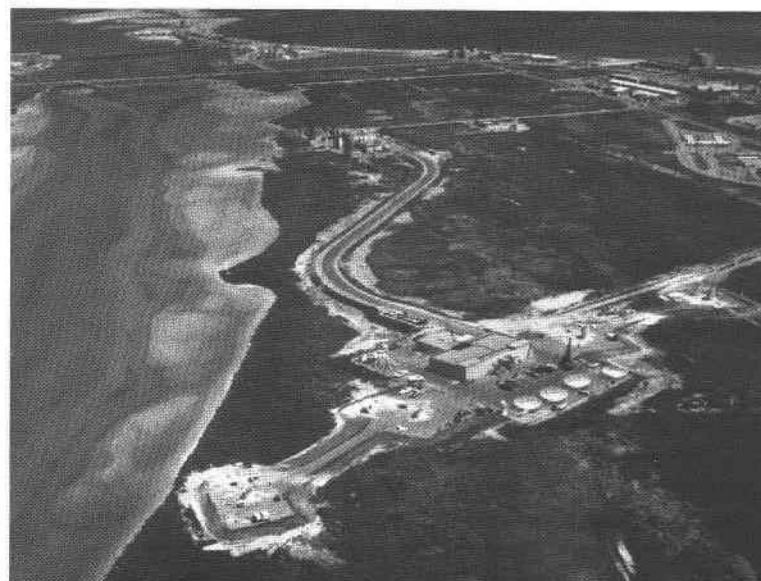
Telemetry Building under construction at Point Mugu (1967).
