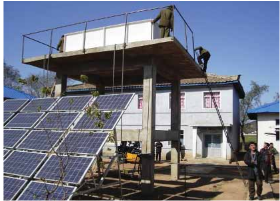
Above: An organic fertilizer plant in North Korea built with NGO assistance. Below: a potable water system where water is pumped by solar power into the elevated tank and then piped into the adjacent school, providing clear, safe, running water.
