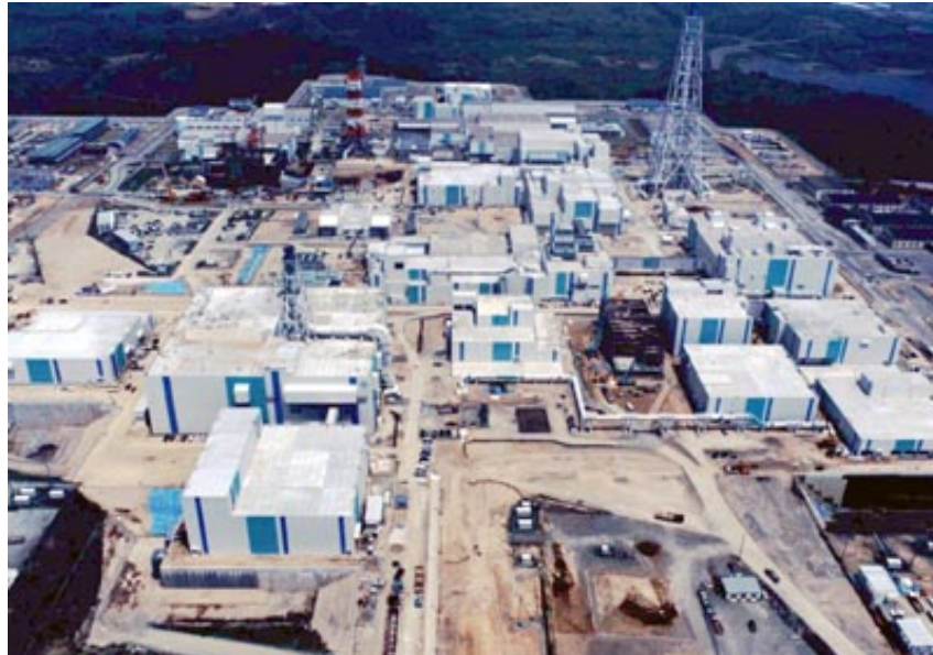
Overview of Construction Site
