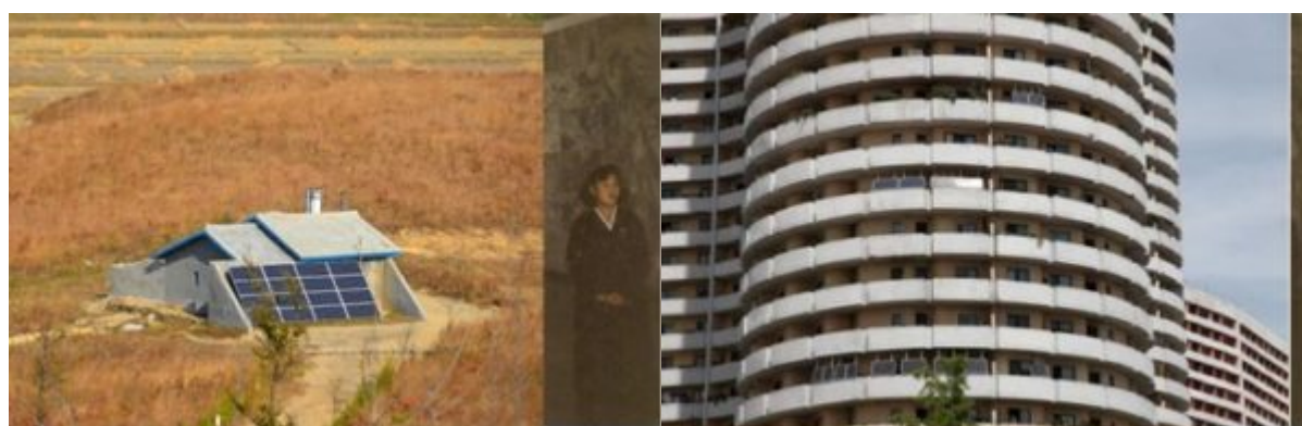
Figure 2-1: Solar PV Panels in Rural and Urban Installations in the DPRK[3]
