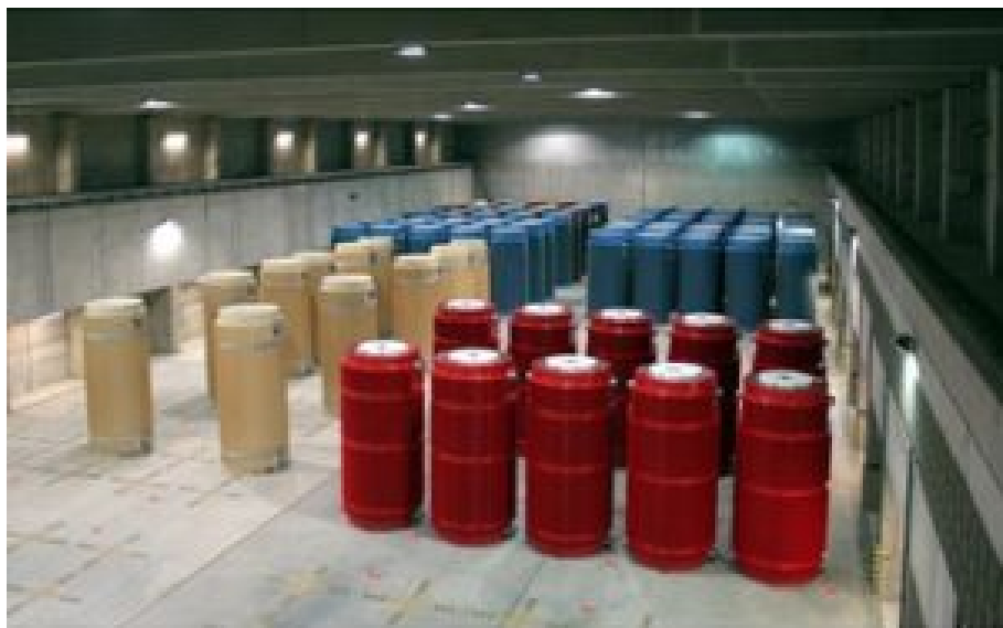
Figure 8: Interim storage facility at Gorleben (Copyright GNS)
