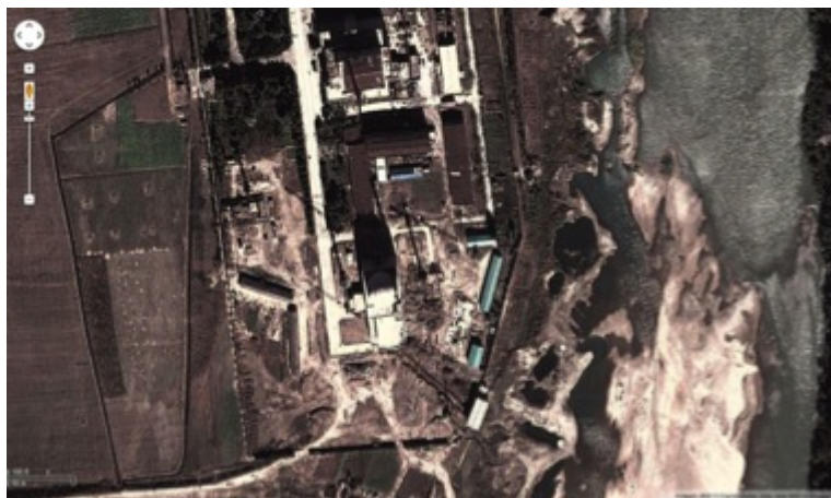
Figure 2-5: Satellite Photo of Yongbyon Reactor, Mid-2013[6]
