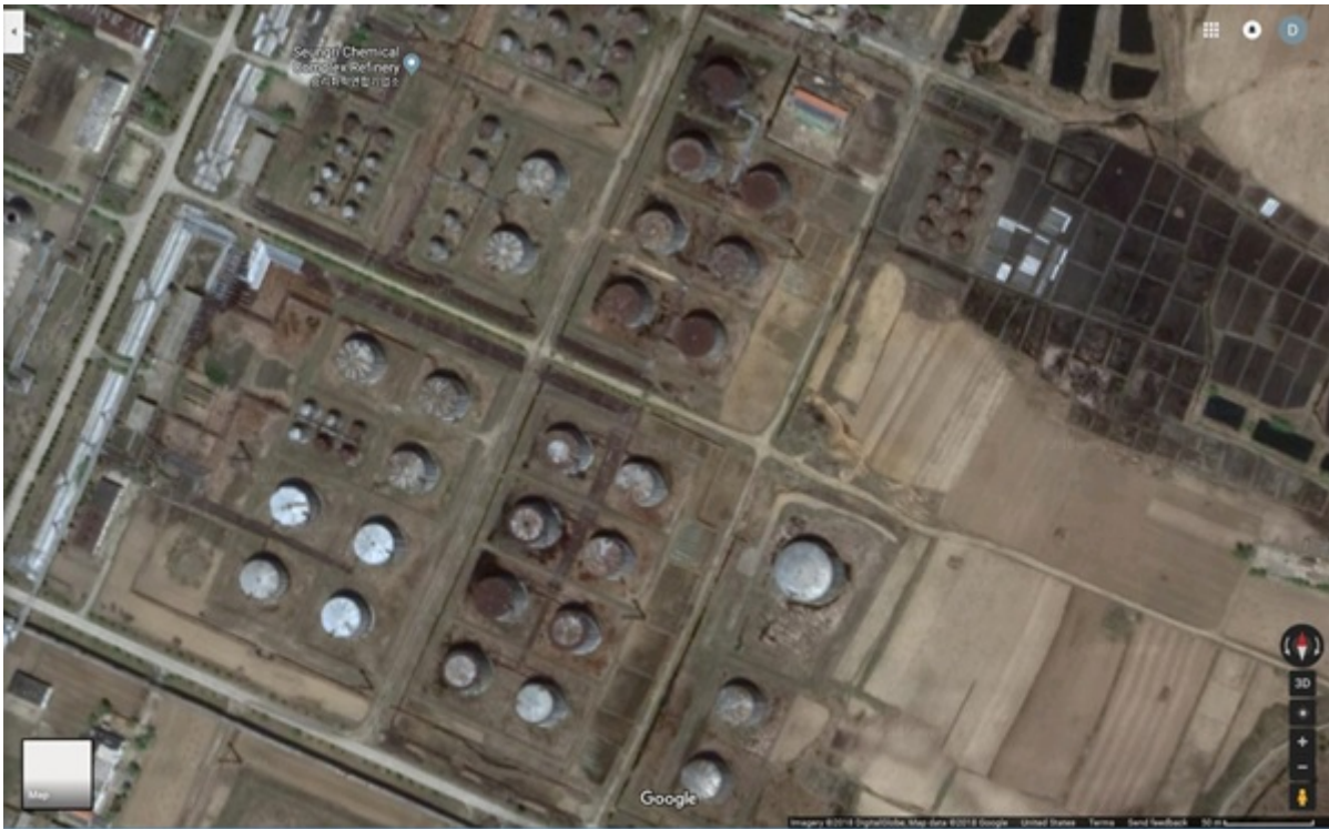
Figure 6: Oil Storage at a Marina near Chongjin
