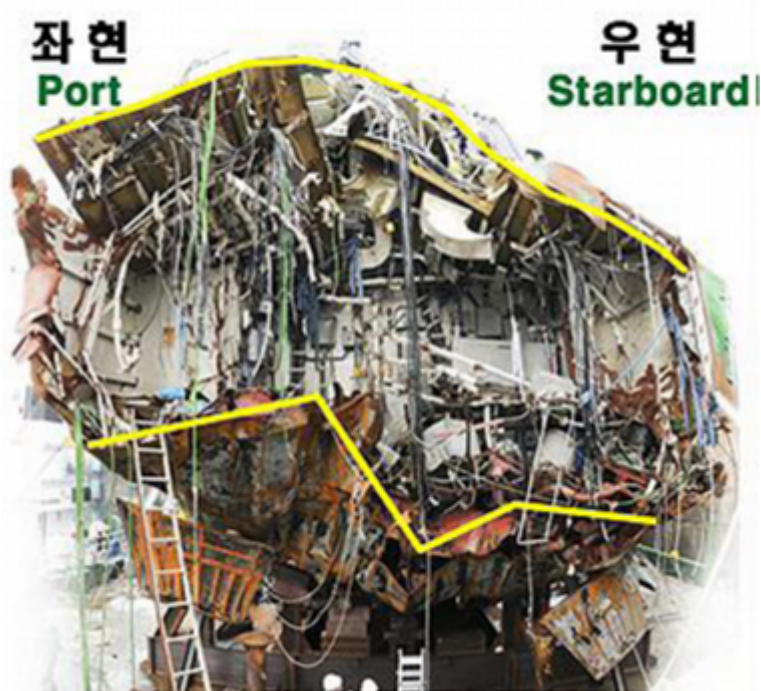
Figure 1. Cheonan’s Damaged Bow
