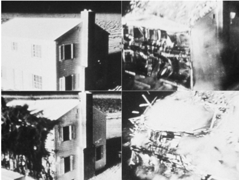
Figure 2. Damage done by 5 psi on a house
