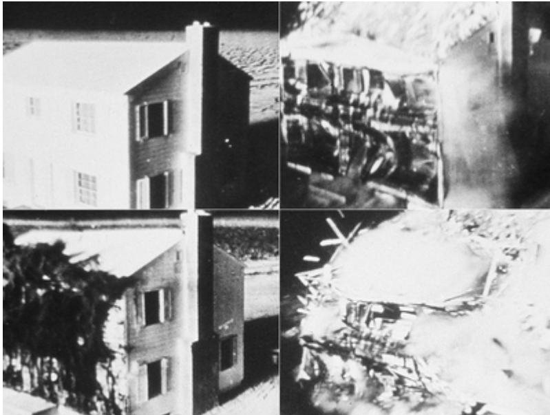
Figure 2. Damage done by 5 psi on a house
