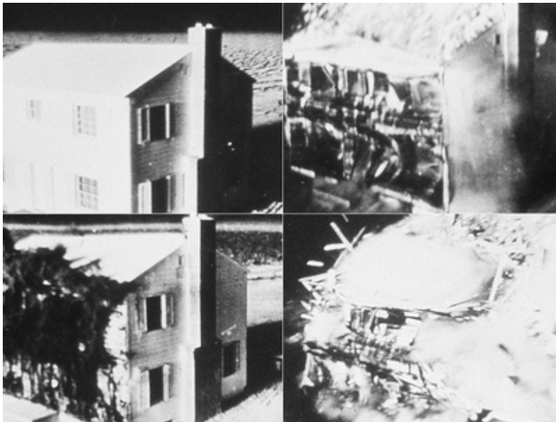
Figure 2. Damage done by 5 psi on a house
