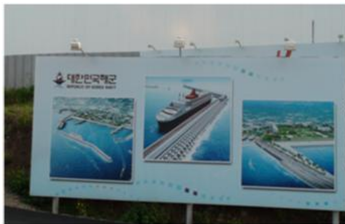
Navy posters at the construction site.
