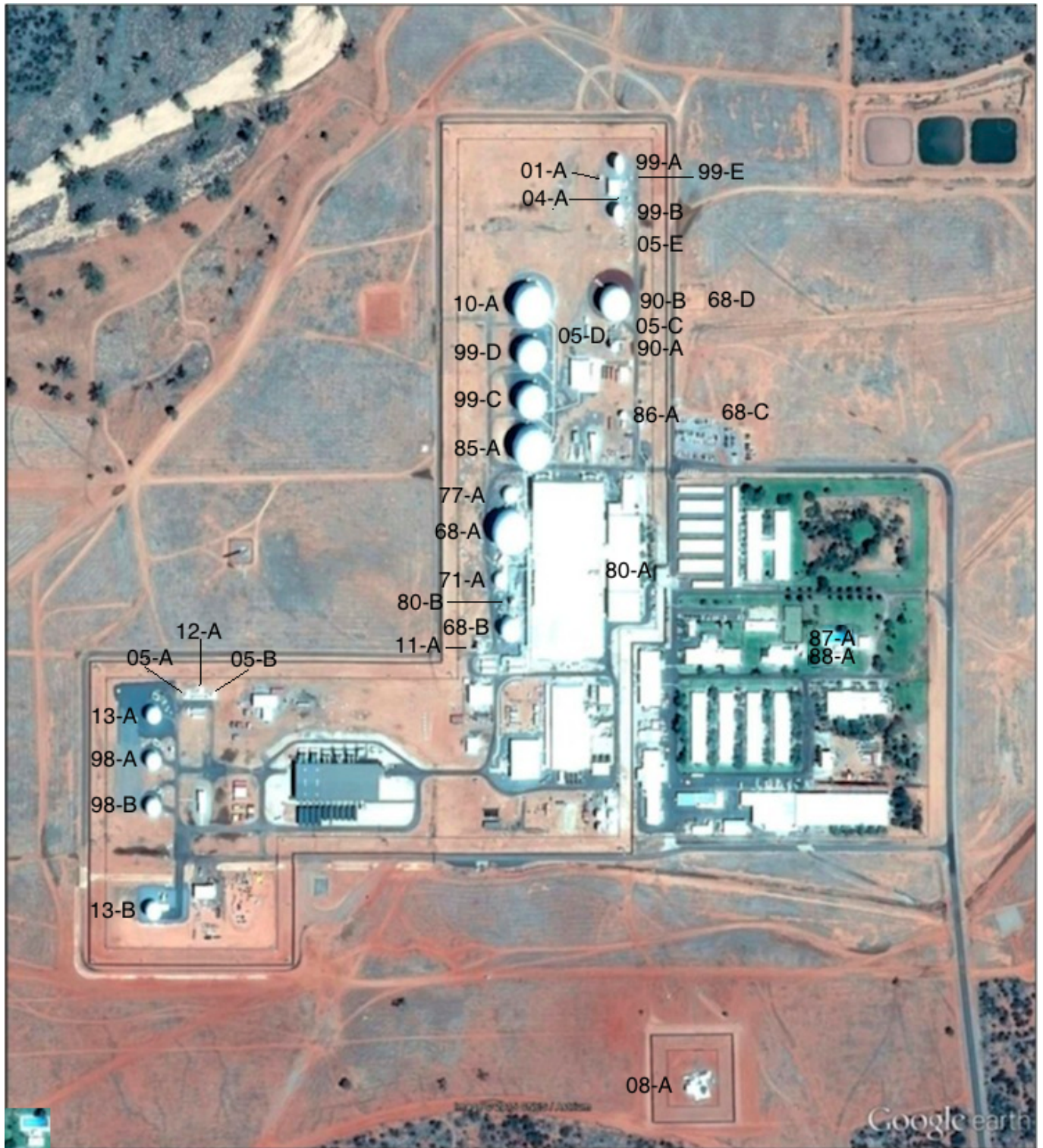
Figure 1. Antenna systems at Pine Gap, Google Earth imagery, 6 November 2015. Note: for antenna identification system see Desmond Ball, Bill Robinson and Richard Tanter, The Antennas of Pine Gap, Nautilus Institute, Special Reports, February 2016.[/caption]
