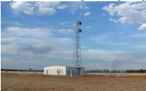
Figure 7: Receiver Site building at Morundah
