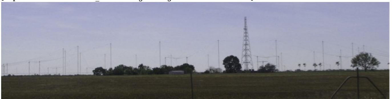
Humpty Doo Transmission Station, transmitter building, central array, and tower, looking west, 2013[/caption]
