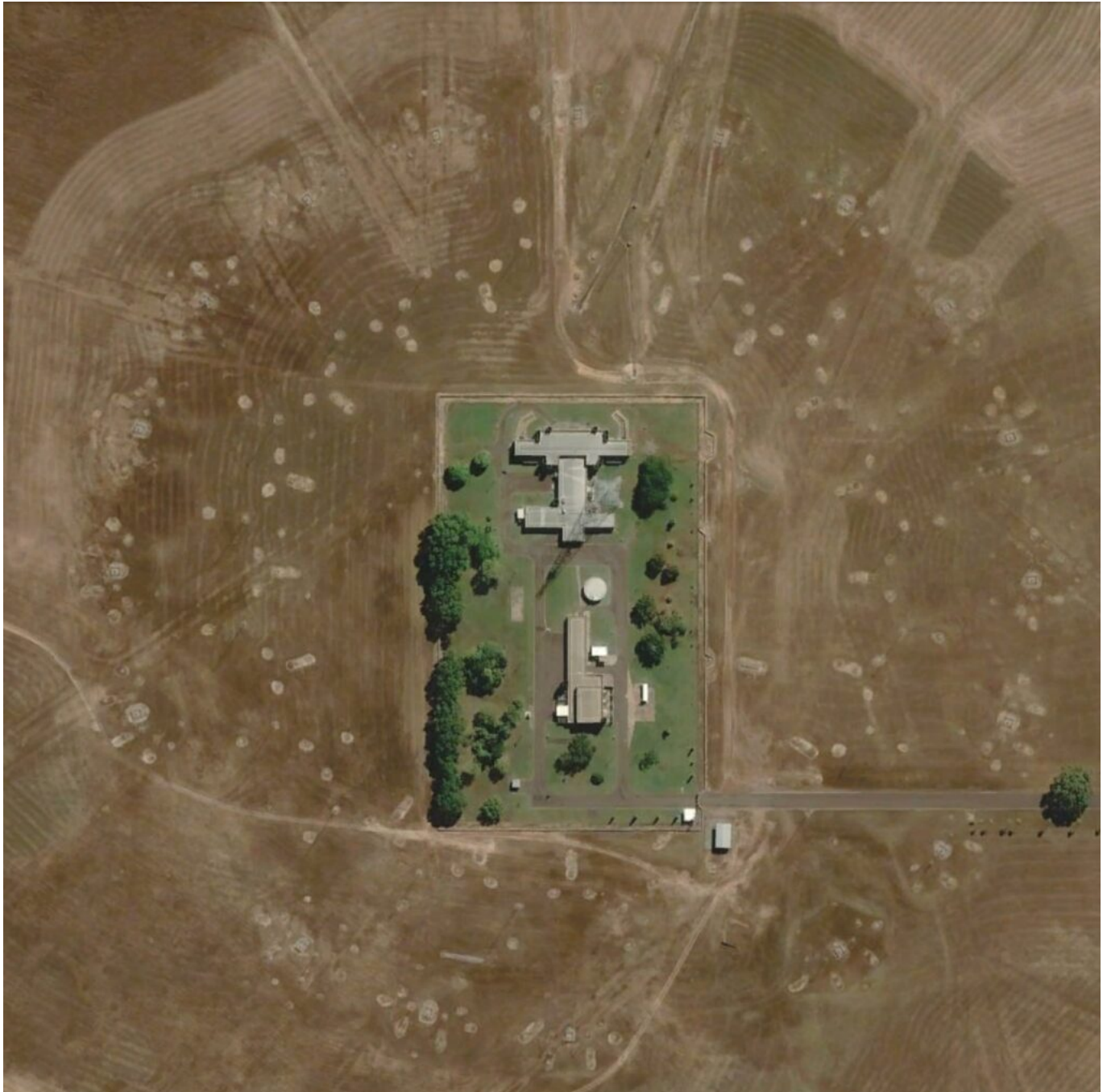
A set of ten smaller antennae are arranged in a further rough circle around the central array.
