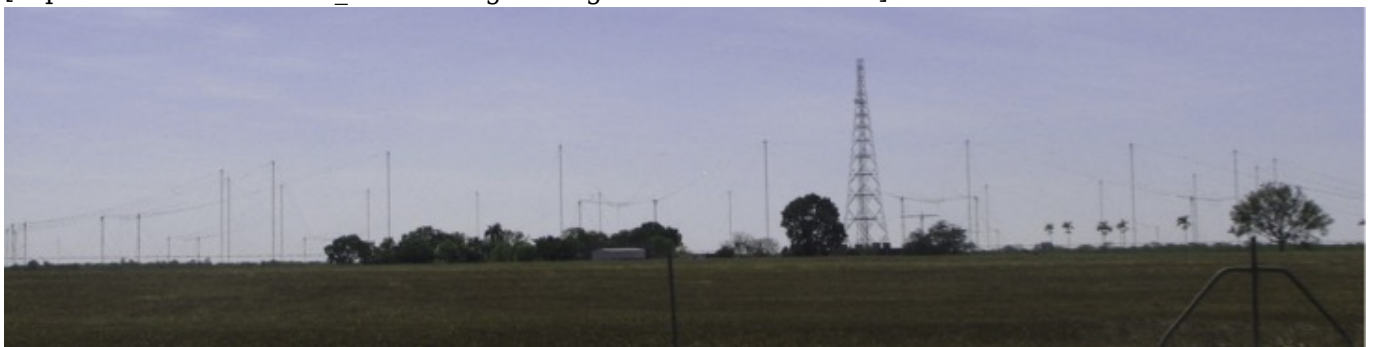
Humpty Doo Transmission Station, transmitter building, central array, and tower, looking west, 2013[/caption]
