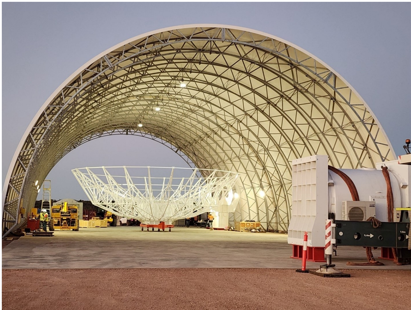
A reflector being assembled in the Antenna Integration Structure (AIS) at DARC Site 1 in Australia. photo credit: Mike Kortum, Four Sea Group Inc. United States Space Force photo by X0813, VIRIN: 250219-X-FC312-1002 .[/caption]
