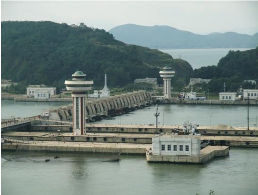
Figure 4-8: Photo of West Sea Barrage, Near Nampo, DPRK 424
