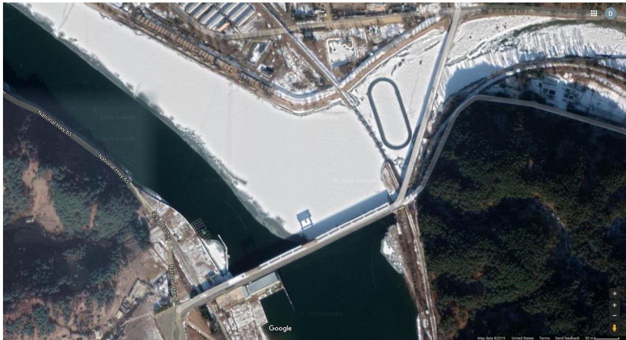
Figure 5-16: Hydroelectric Plant on the Chongchon River 555
