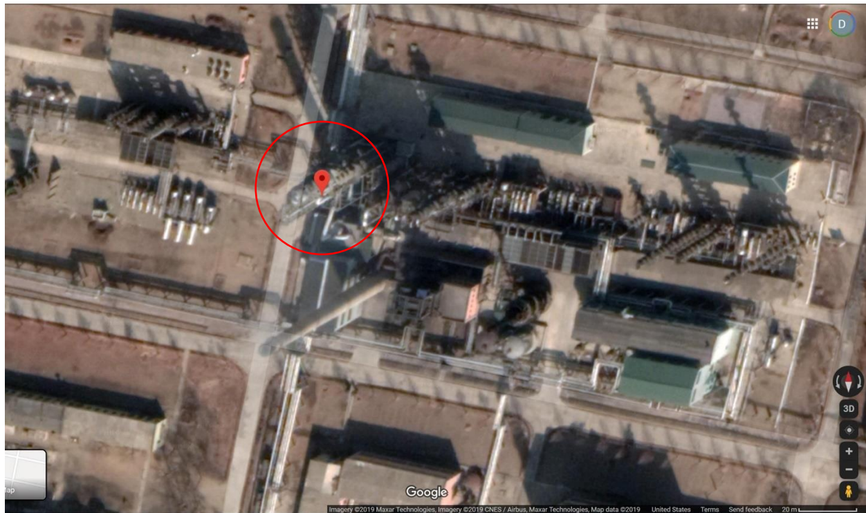
Figure 6-11: Likely Catalytic Cracking Unit Installed at Ponghwa Chemical Factory
