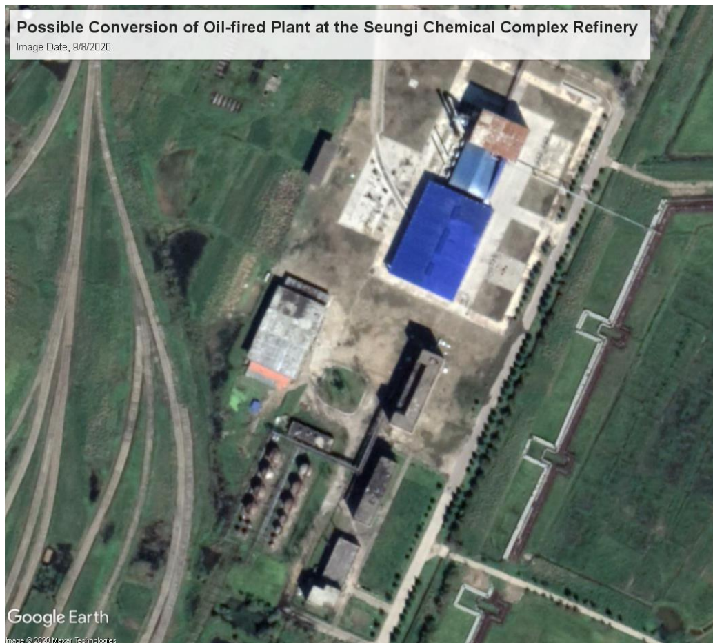
Figure 5-10: Satellite Photo of the Possible Ongoing Conversion of the HFO-fired Power Plant at Sonbong as of September 2020 (Source, Google Earth Pro)
