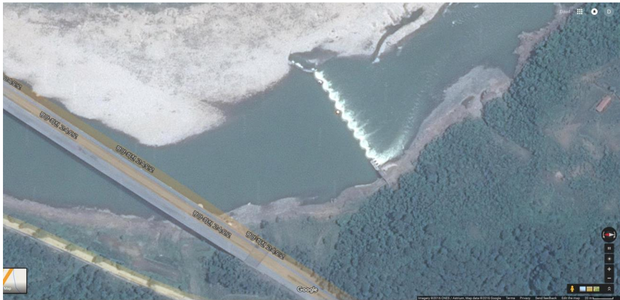
Figure 5-14: Satellite Photo of Probably Small Hydroelectric Plant (name unknown) Downstream from Huichon #2 Hydroelectric Power Plant, Apparently in Operation as of Late 2015 or Early 2016 (Source, Google Maps)
