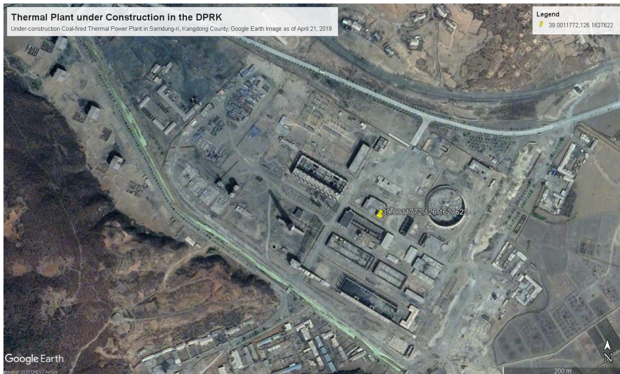
Figure 5-9: Satellite Photo of the Under-construction “Kangdong” Thermal Power Complex in as of Spring 2019 (Source, Google Earth Pro) 532
