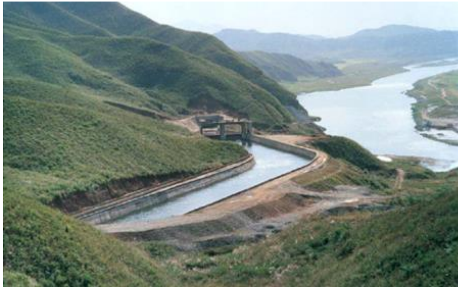
Figure 5-45: Natural-flow Irrigation Waterway in the DPRK Completed Circa 2004-2005 640
