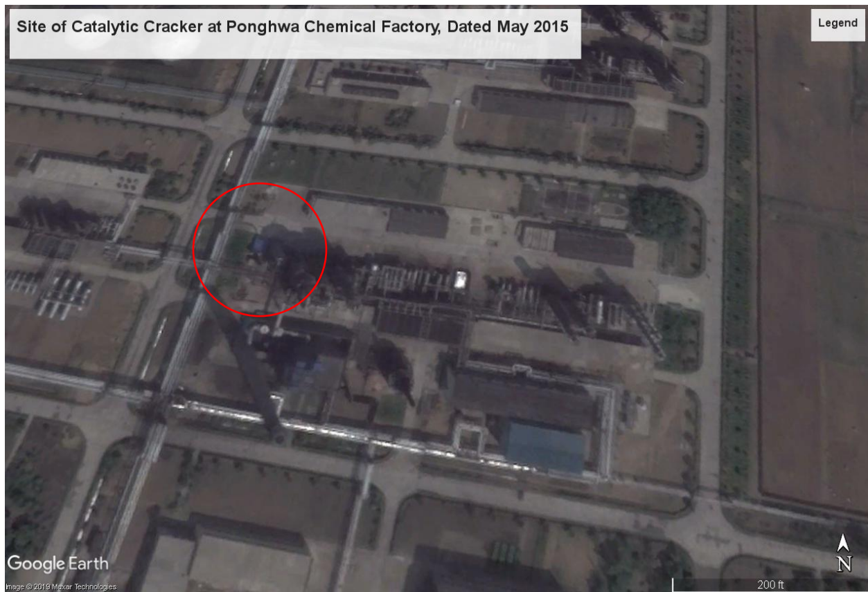
Figure 6-12: Site of Future Catalytic Cracking Unit as of May 26, 2015 680
