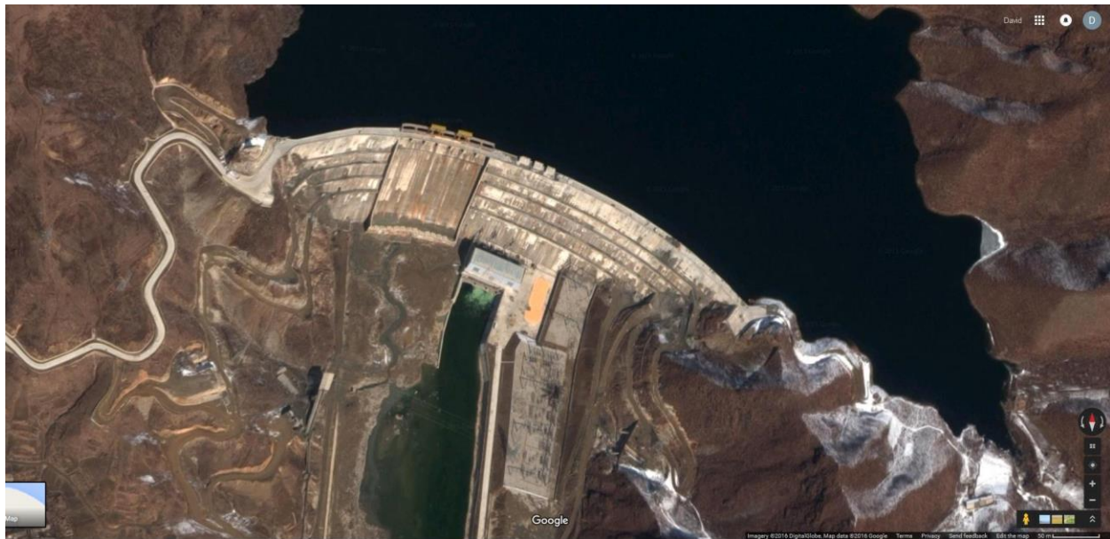
Figure 5-13: Satellite Photo of Huichon #2 Hydroelectric Power Plant, Apparently in Operation as of Late 2015 or Early 2016 (Source, Google Maps)
