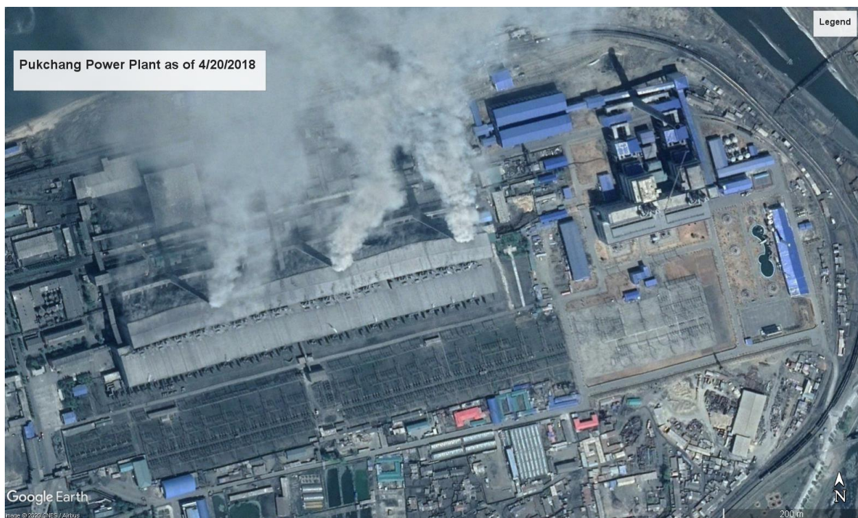
Figure 5-8: Satellite Photo of the Pukchang (or Bukchang) Thermal Power Complex in Operation as of Spring 2019 (Source, Google Earth Pro) 531
