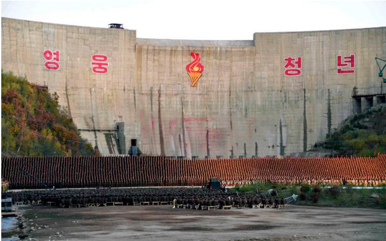
Figure 5-15: Mount Paektu Power Station Dam at Dedication Ceremony in October, 2015 554
