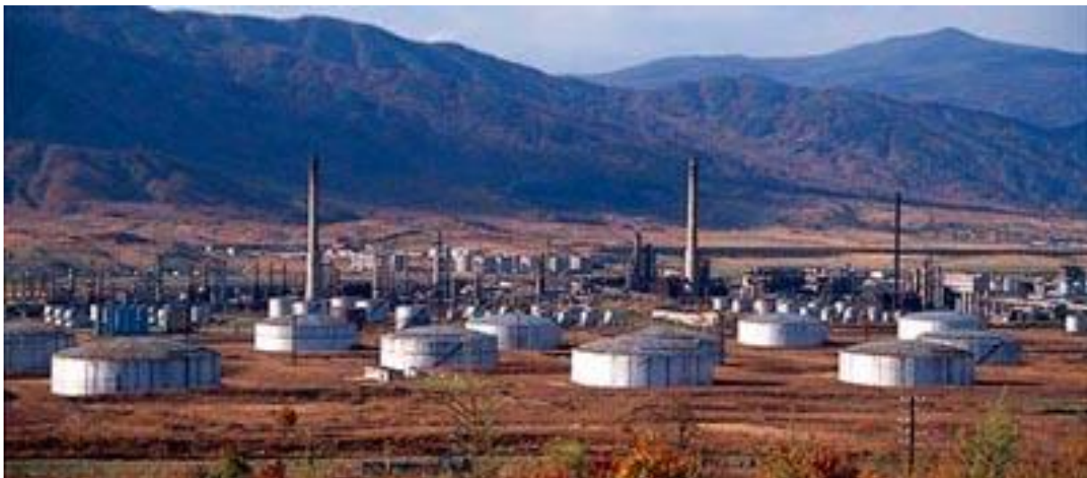
Figure 2-8: Photo of Sungri Chemical Plant Oil Refinery
