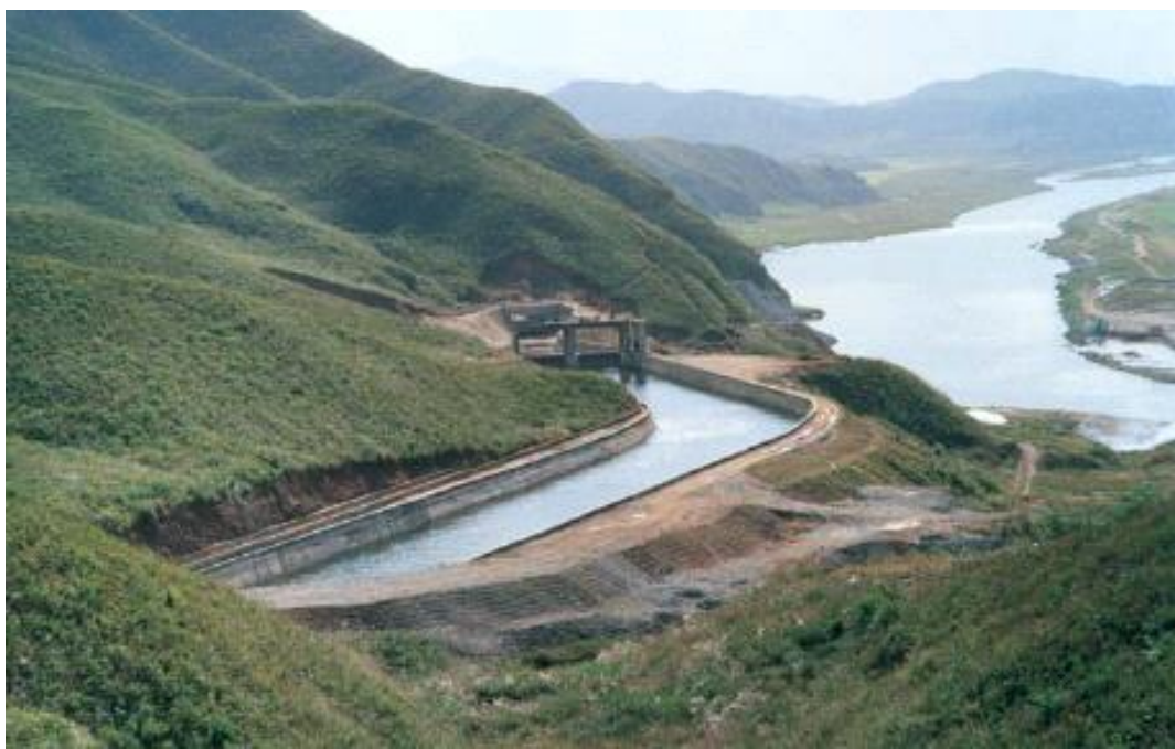
Figure 3-10: Natural-flow Irrigation Waterway in the DPRK Completed in the Early 2000s 339
