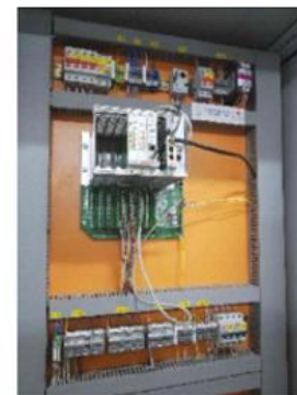
c. Existing RTU cabinet
