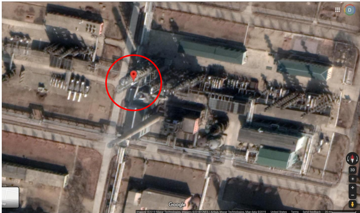
Figure 11: Likely Catalytic Cracking Unit Installed at Ponghwa Chemical Factory
