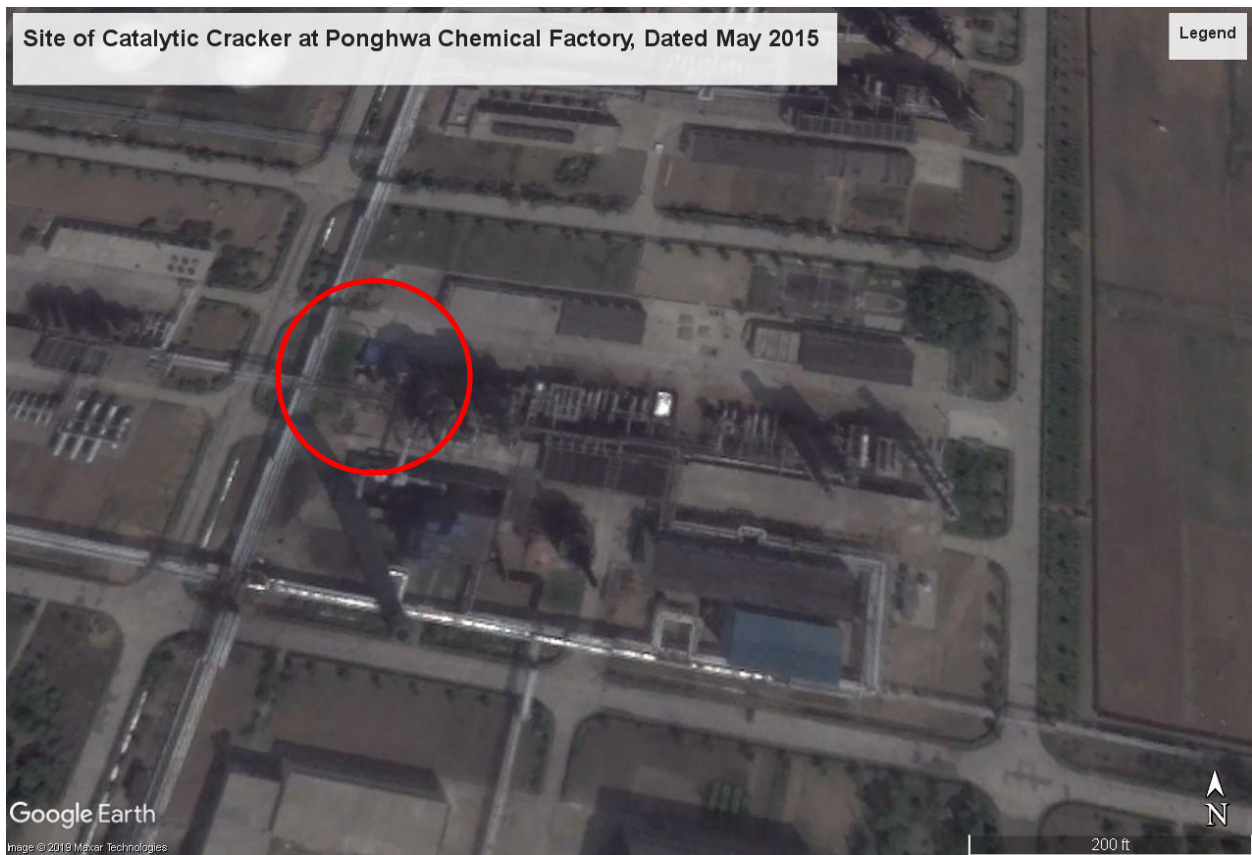
Figure 12: Site of Future Catalytic Cracking Unit as of May 26, 2015 20
