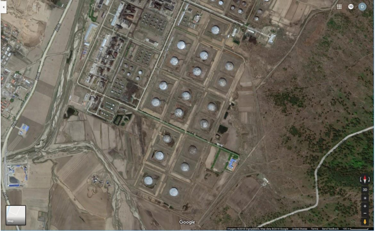
Figure 5: Two Views of Specific Tank Locations at the Seungri Chemical Complex
