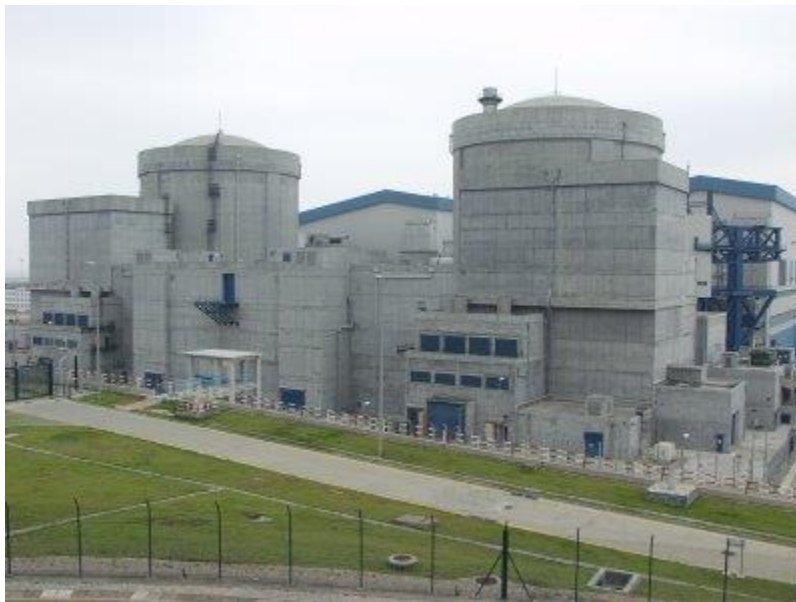
Figure 2-12: Photo of Ling' Ao Phase I Nuclear Power Units 31
