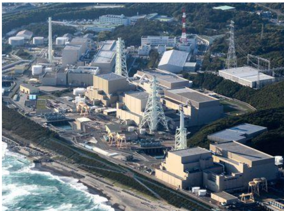
Figure 2-24: Aerial Photo of Hamaoka Nuclear Power Plant 40
