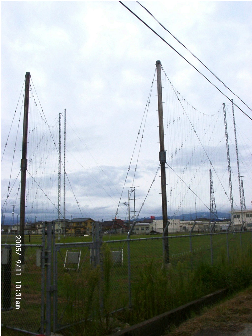
Plate 54 HF vertical curtain arrays, DIH SIGINT station, Kobunato, 11 September 2005
