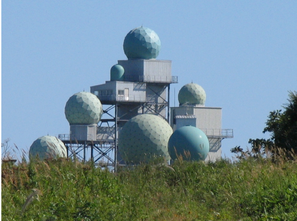
Plate 32 J/FLR-2 system, JASDF SIGINT station, Nemuro, from the north side, 9 September 2005
