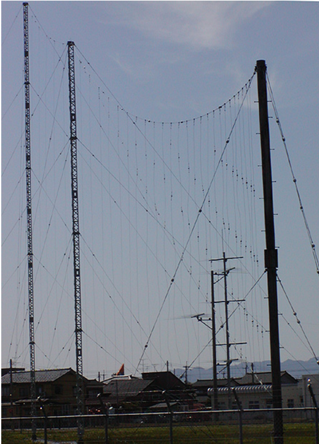
Plate 55 HF vertical curtain arrays, DIH SIGINT station, Kobunato, April 2007
