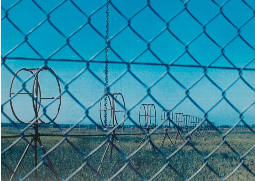
Plate 57 16-element Hermes double-loop antenna array, DIH SIGINT station, Kobunato, May 1988. (Removed soon thereafter)
