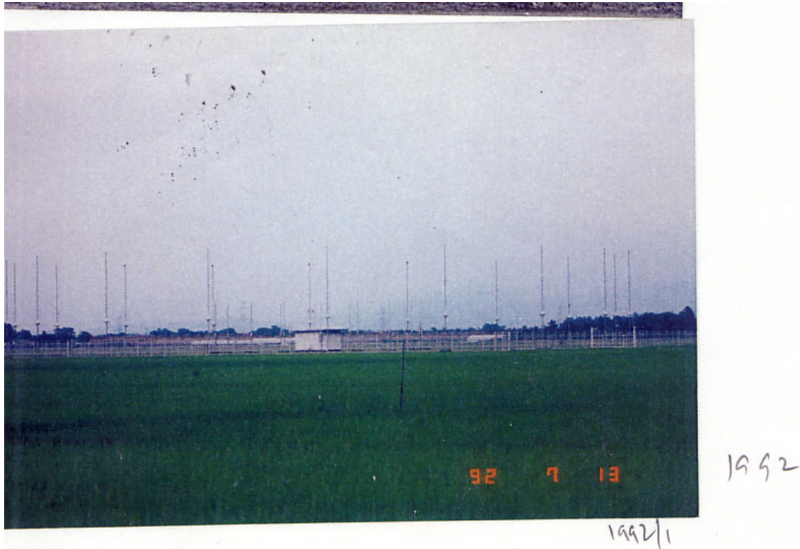
Plate 60 36-element HF DF CDA , DIH SIGINT station, Kobunato, 13 July 1992
