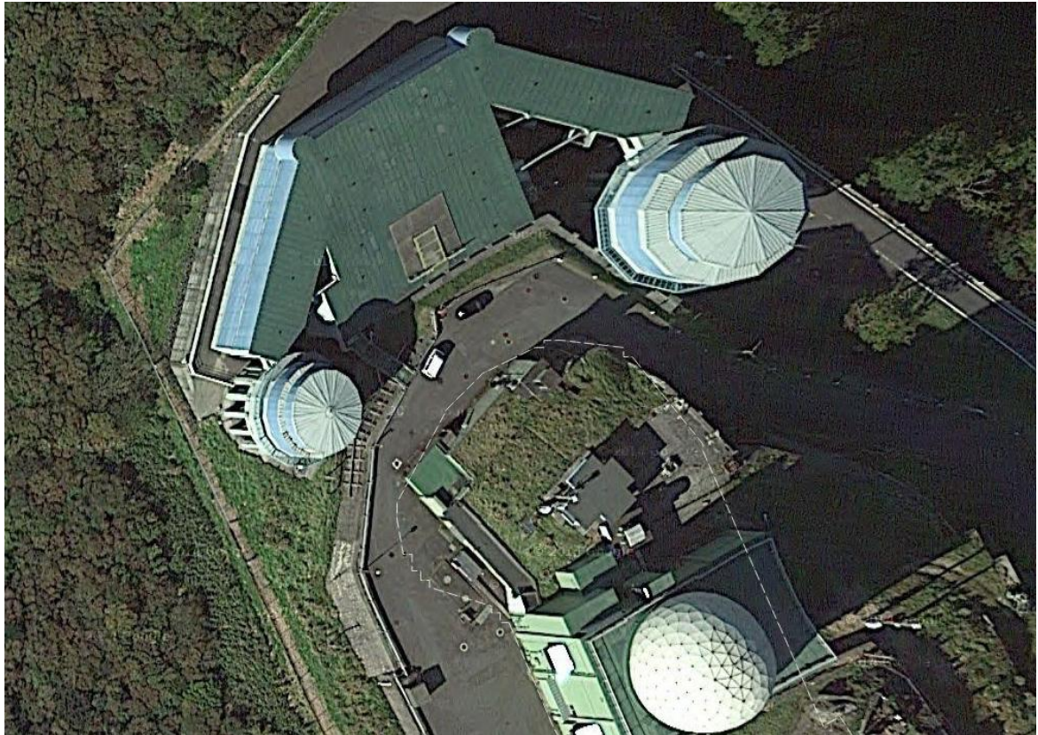
Plate 104 J/FLR-4 SIGINT system (with J/FPS-3 JADGE radome in foreground), JASDF JADGE station, Seburi-yama, GoogleEarth imagery, 16 October 2014
