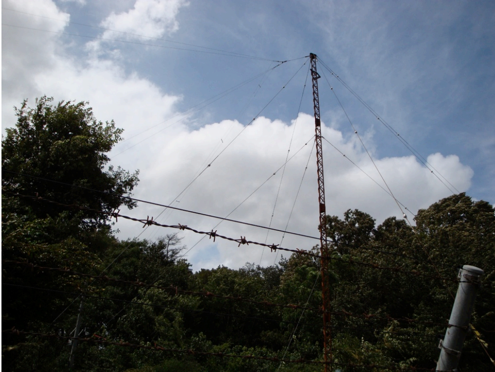
Plate 65 HF antenna (East side of the compound), JGSDF/DIH SIGINT station Ooi, 3 September 2011
