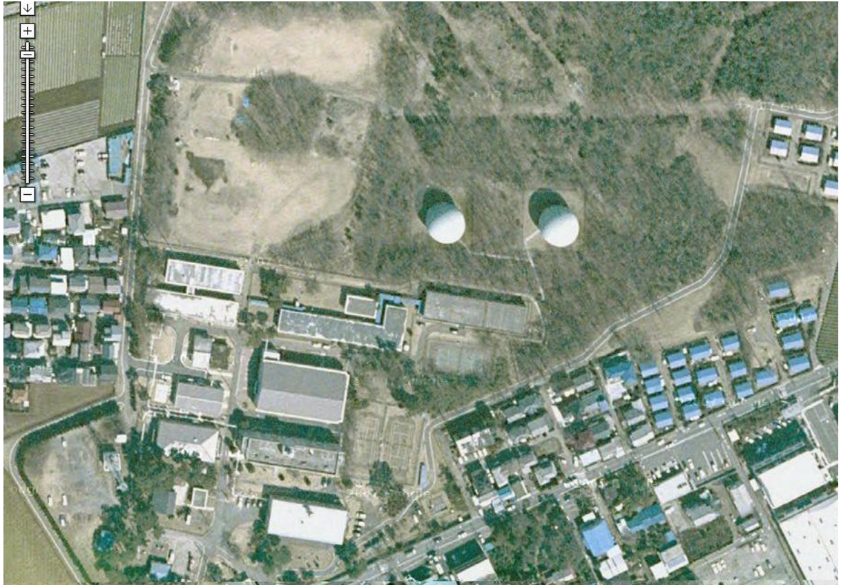
Plate 64 JGSDF/DIH SIGINT station Ooi, (with two 20-metre radomes), GoogleEarth imagery, c2006
