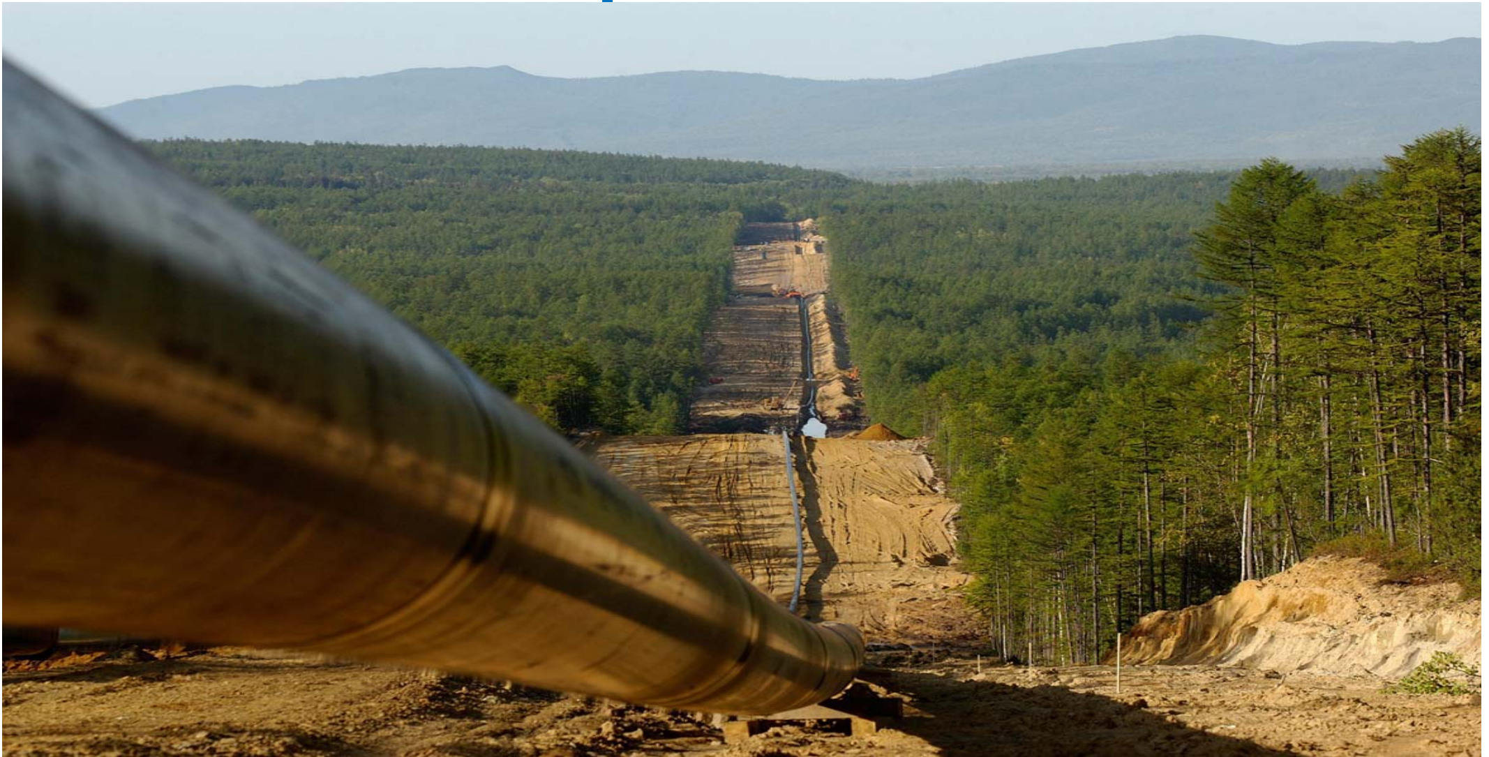
Pipelaying in Onor District
