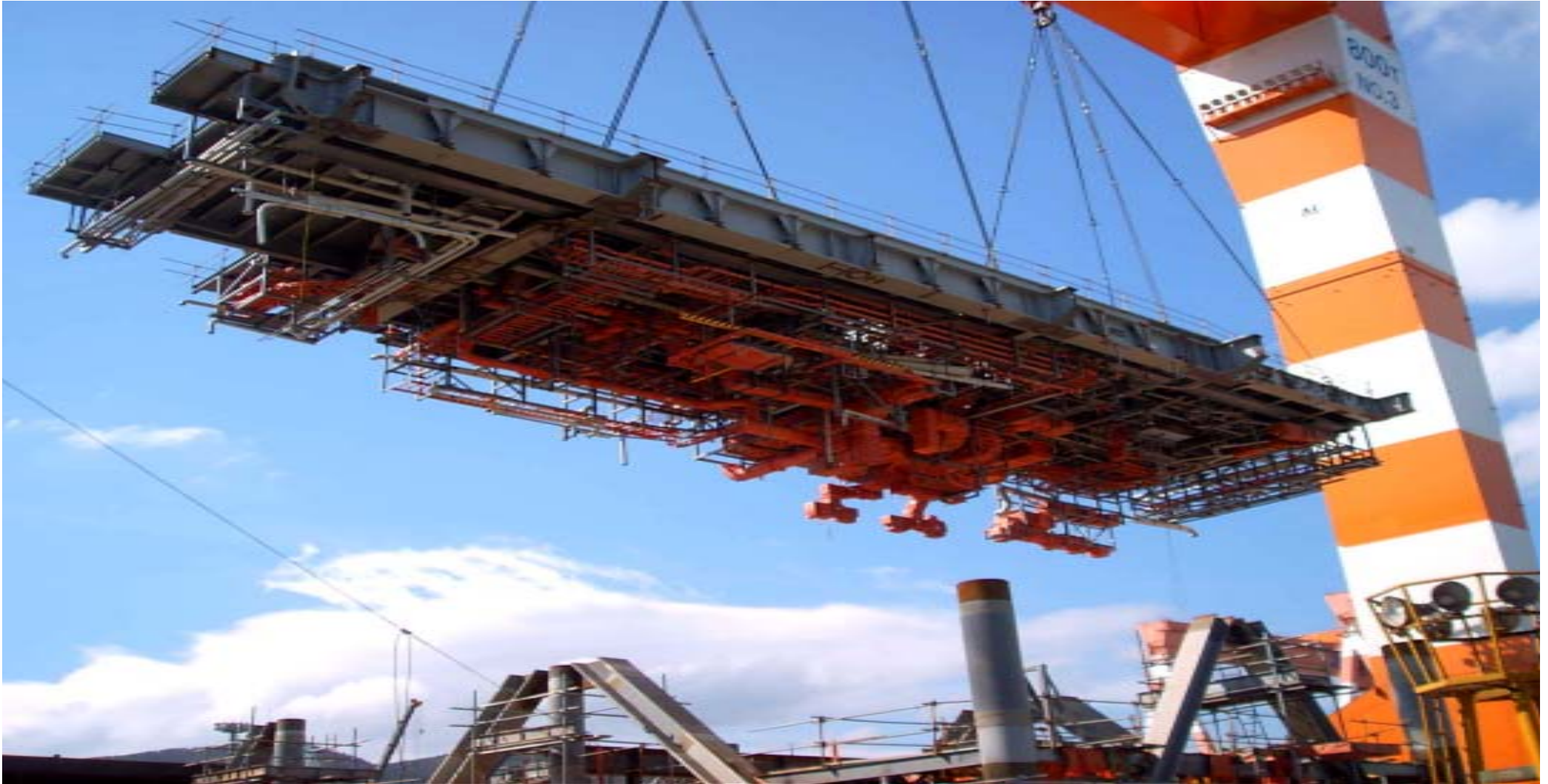
Installation of UD40 with underdeck outfitting in place
