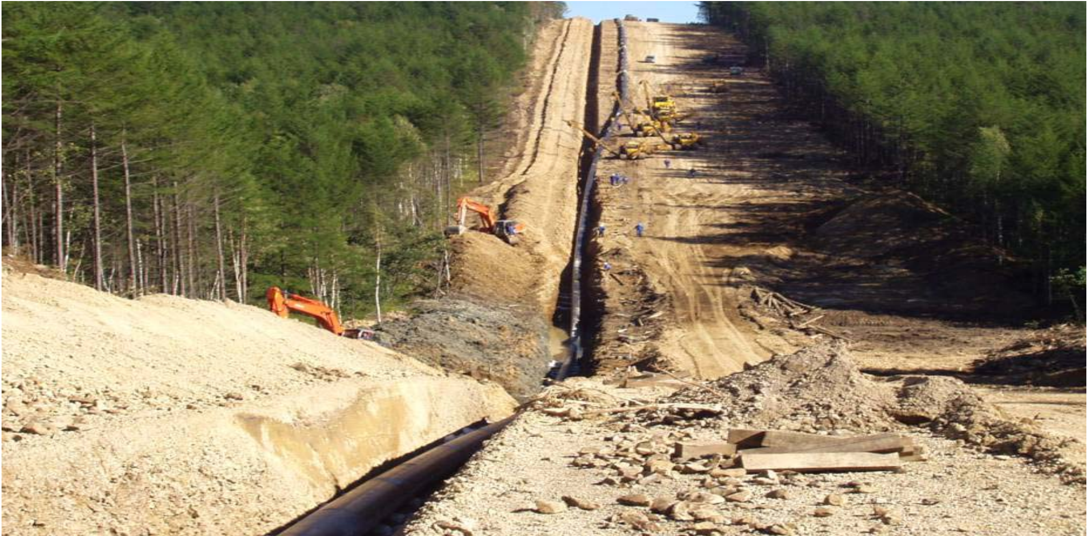
Lowering at KP 589
