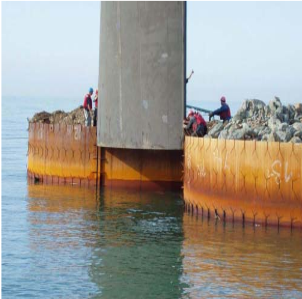
Installing first MOF insert
