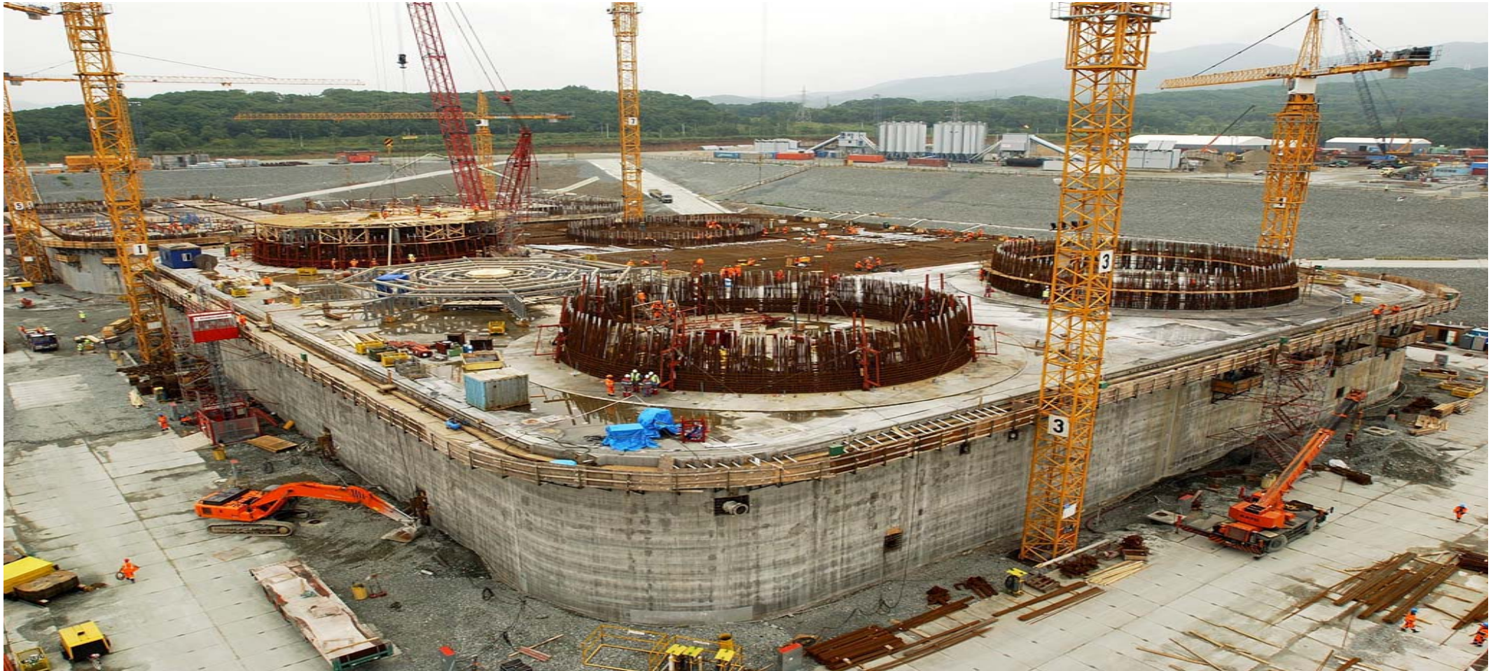
GBS Concrete Base
