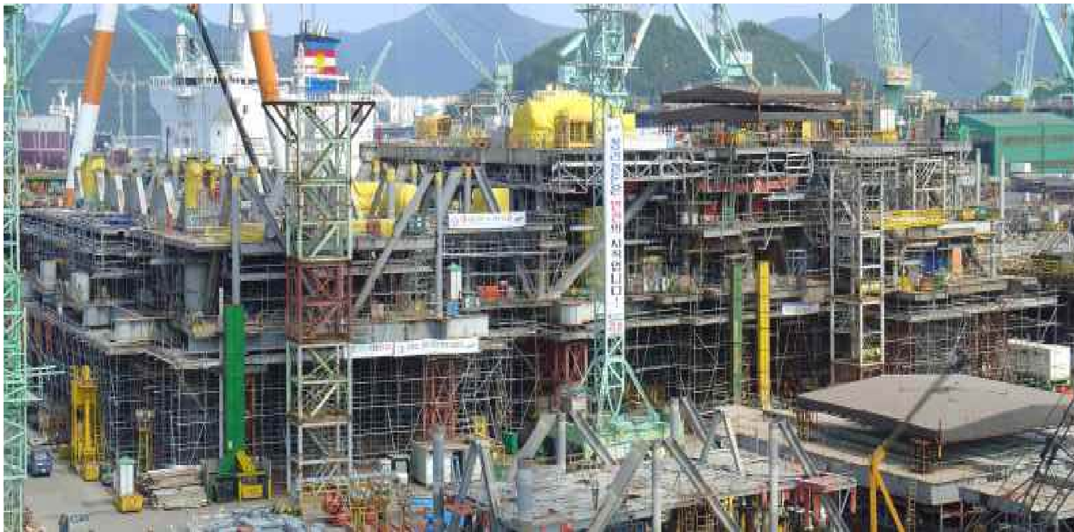
Upper Deck Block UD30 Installed
