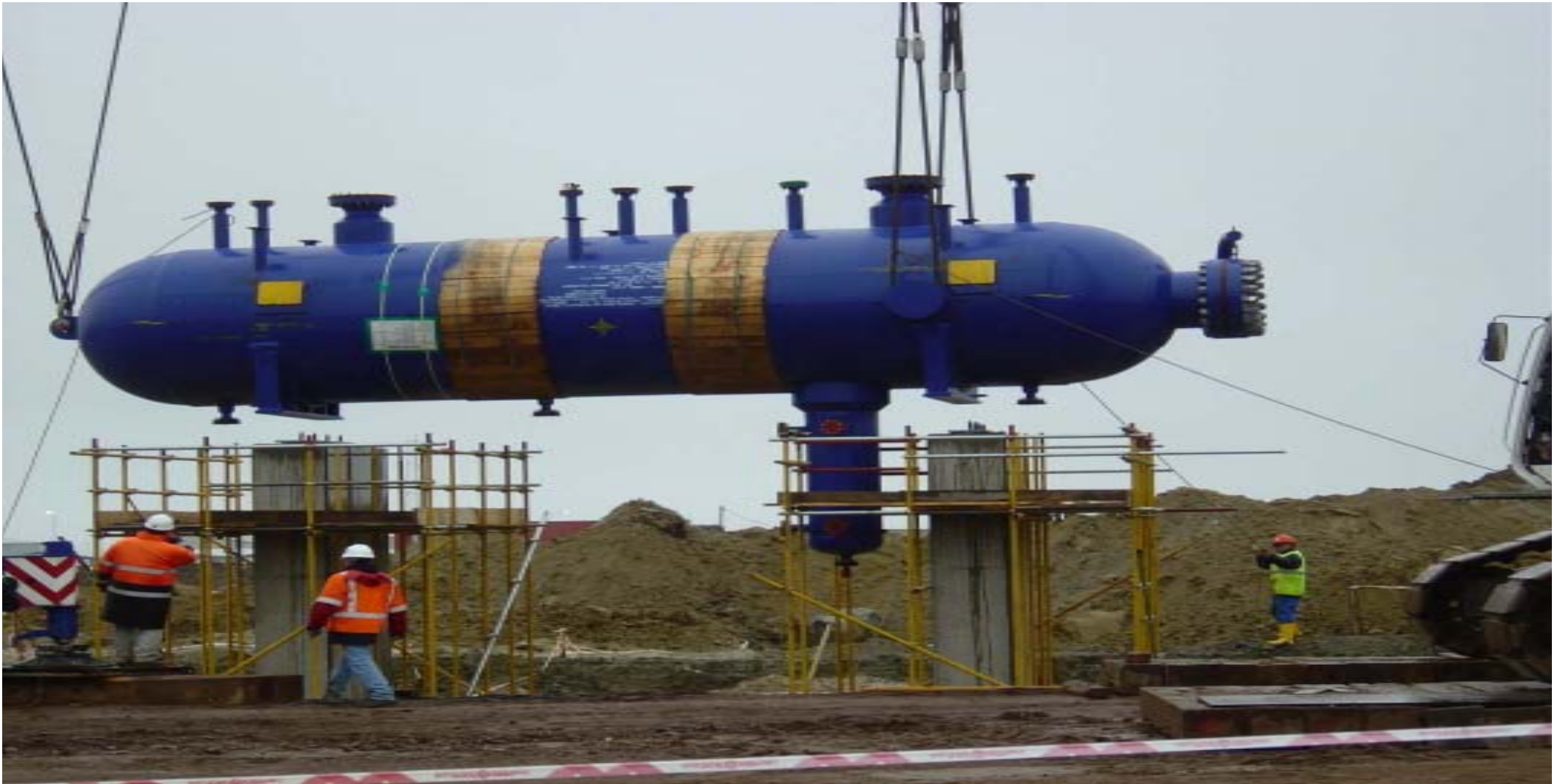
Parking Loop Vessel – Loaded onto Foundations
