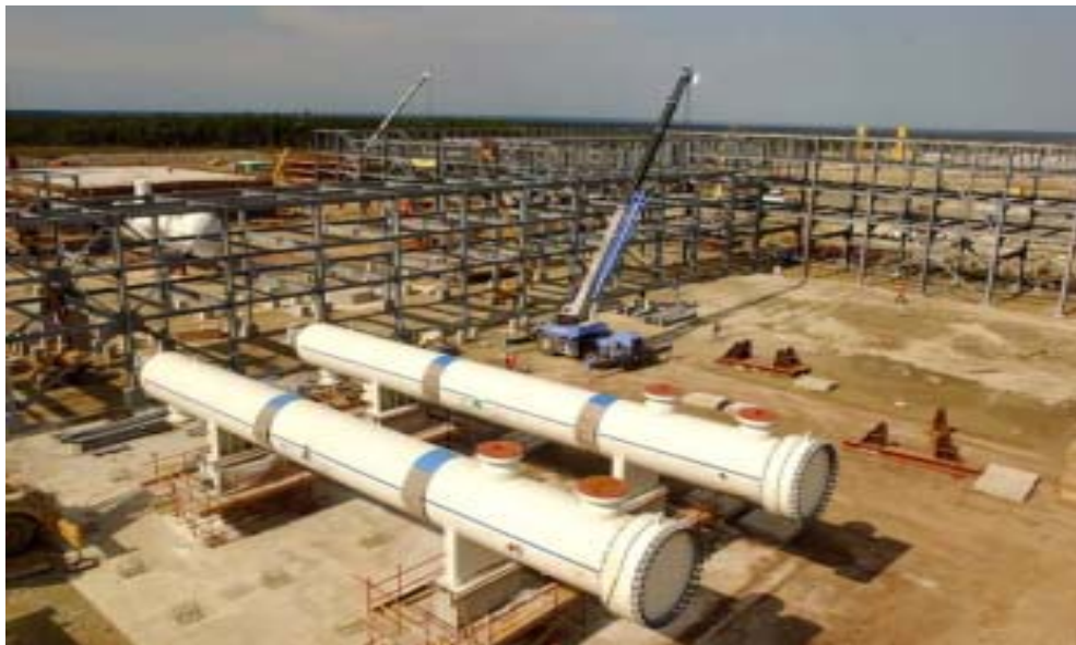
Gas/Liquid Exchanger onto Foundations
