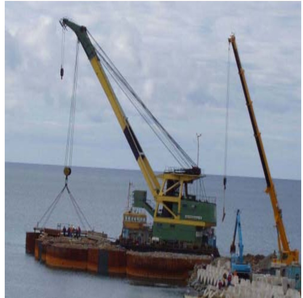
Installing fourth MOF cell
