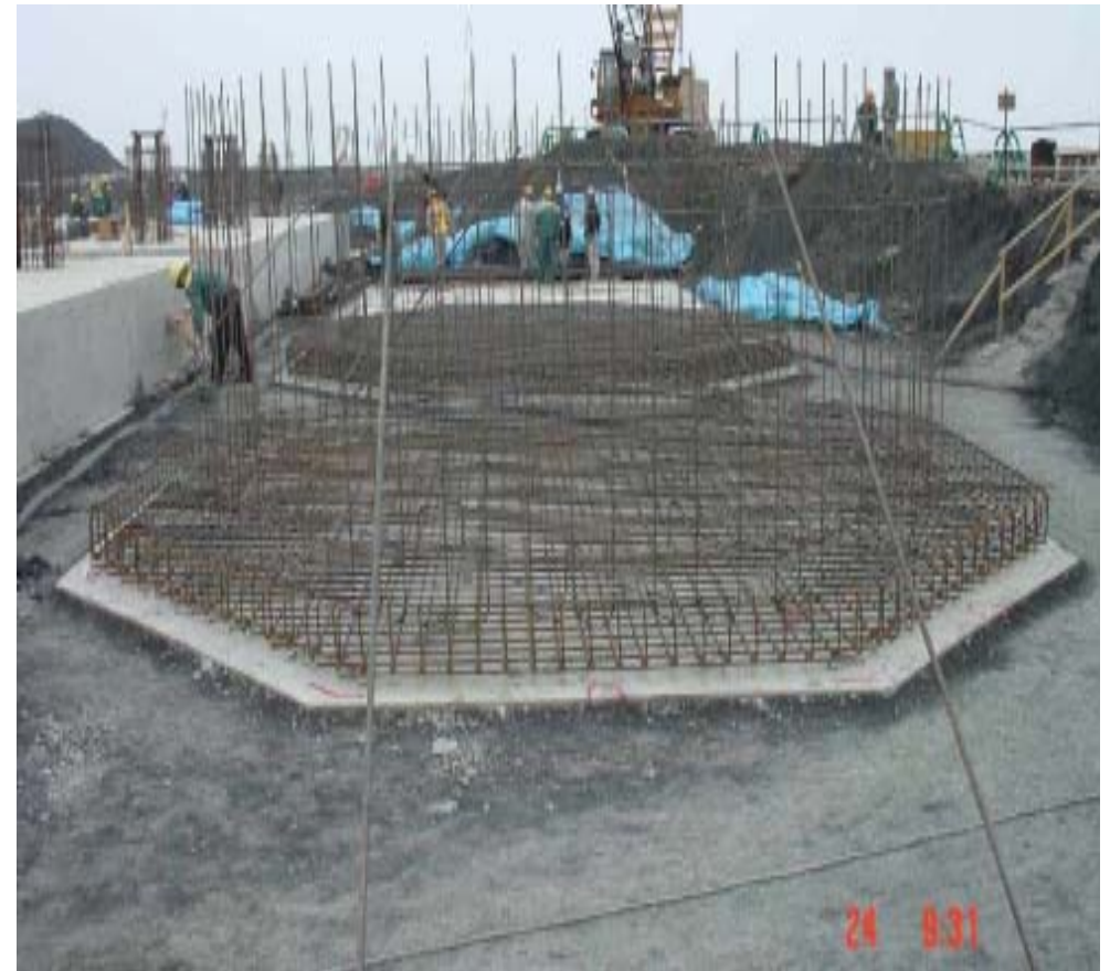
Process Train-1 C-1301 ABC Rebar Installation
