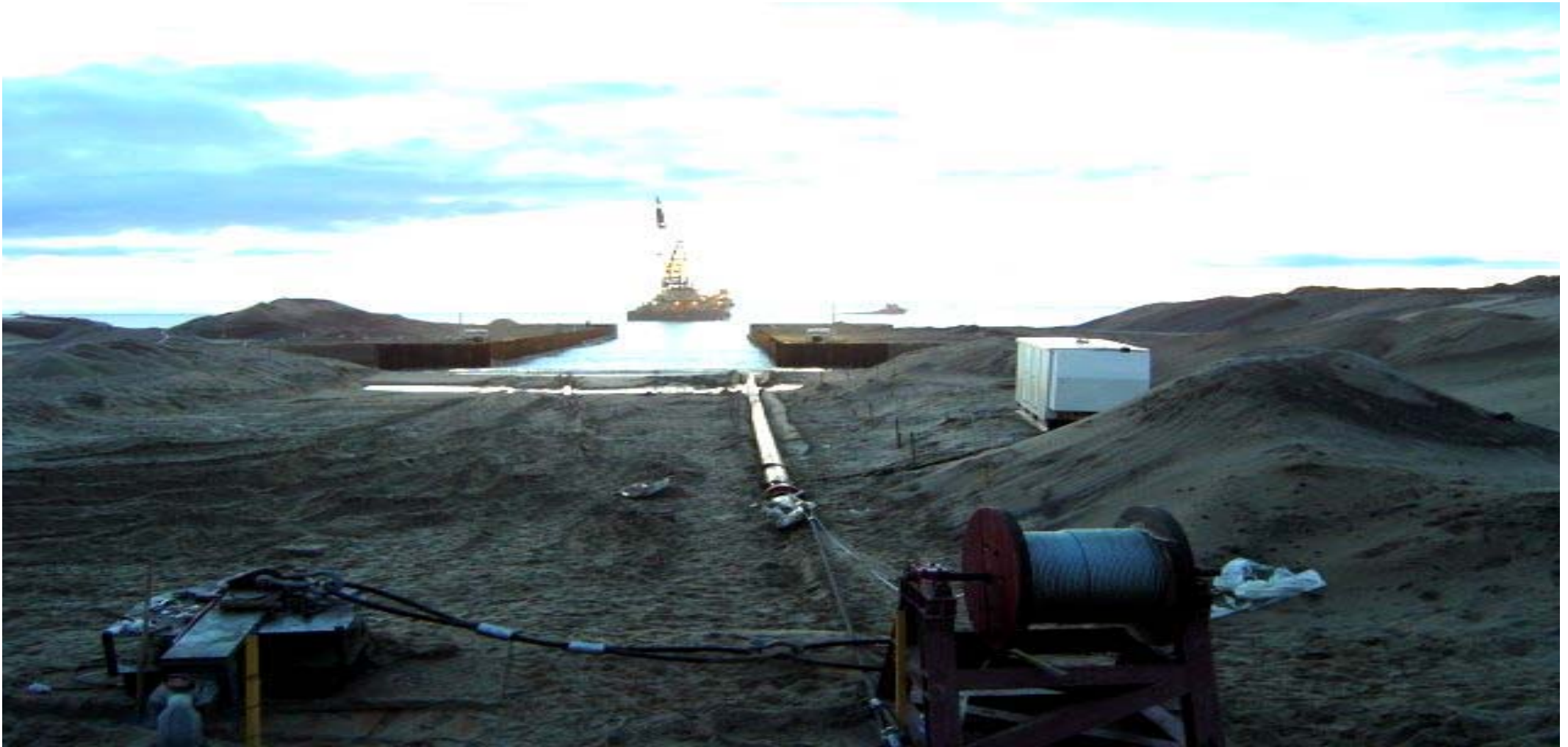
Cable Casing Pulled to Shore
