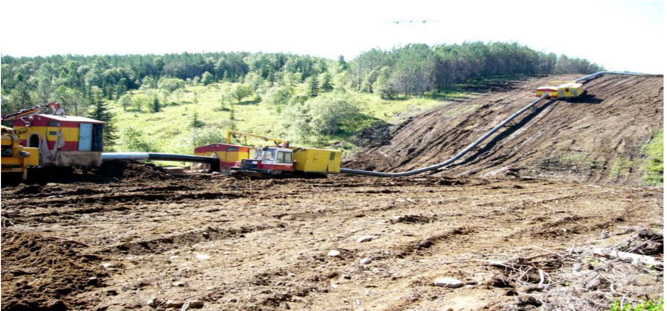
Welding at KP 336
