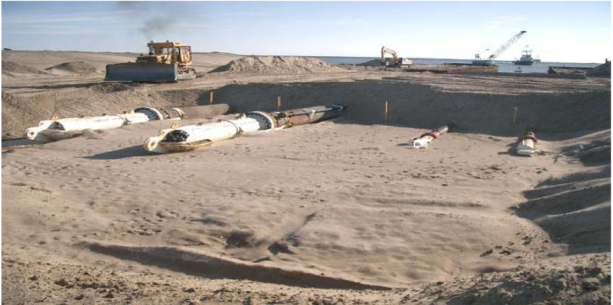
Lunskoye Landfall – Cofferdam with Pull-heads
