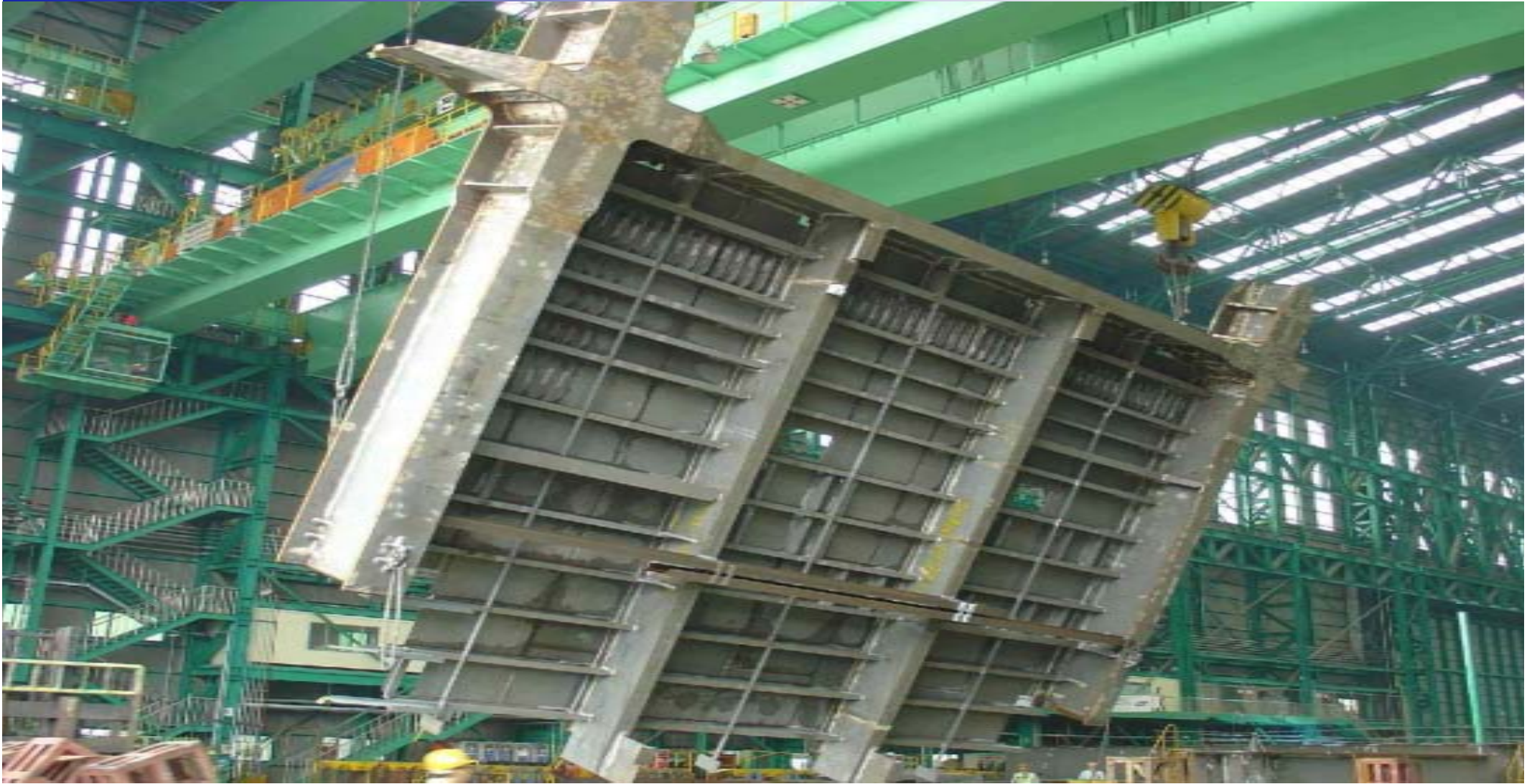
PAB Lower Deck Block LD 21 – Turn Over
