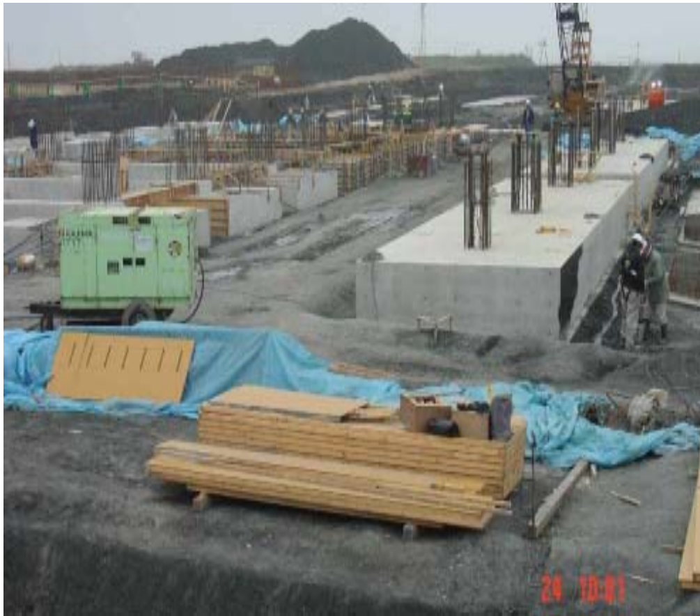
Process Train-1 PR-101 Base Concreting Block-1
