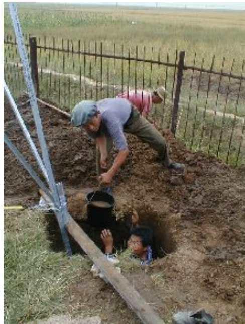
Digging Holes for Windmill Construction
