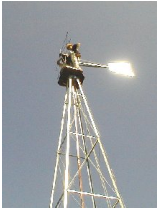
Installing Tail on Windmill
