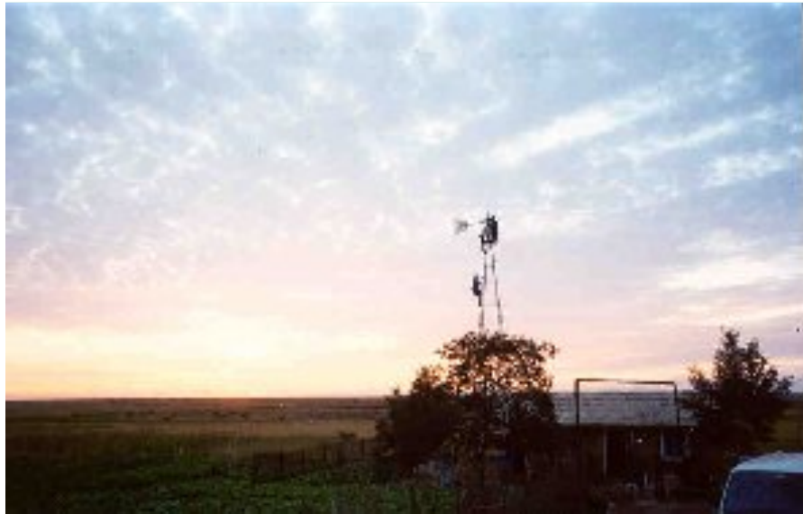
Team Finishing Work on Windmill as Sun Sets over Unhari
