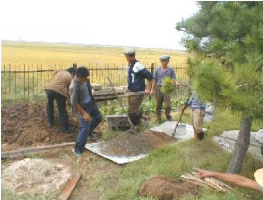
Mixing the Concrete
