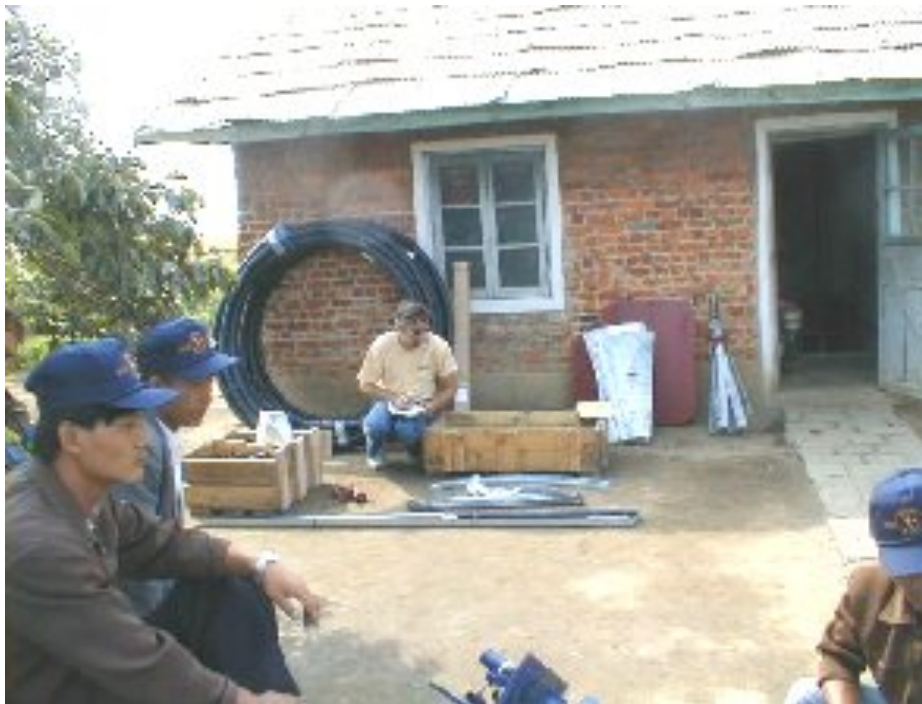
Equipment for Windmill Installation
