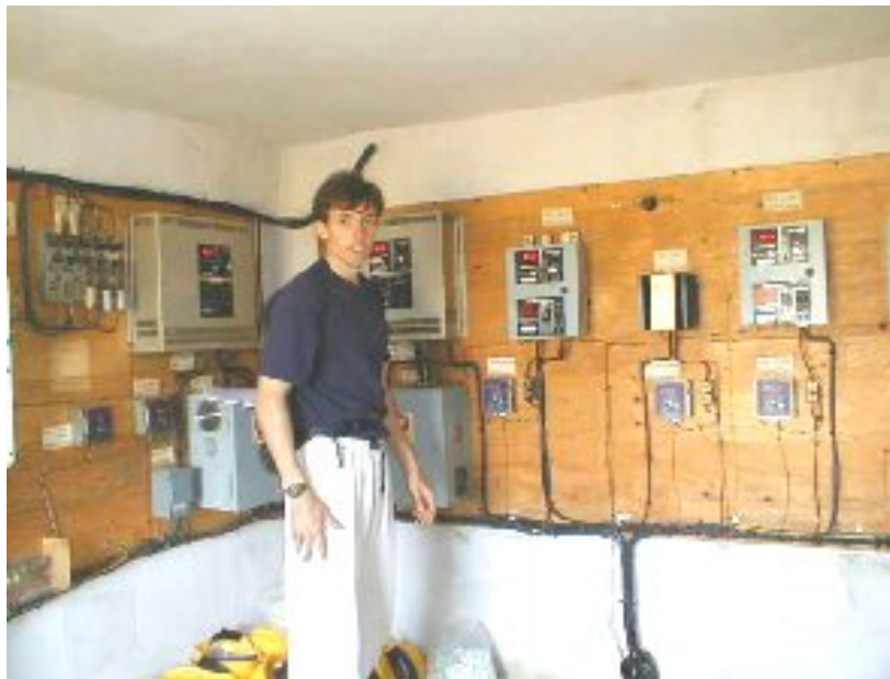
Chris Greacen in the Powerhouse
