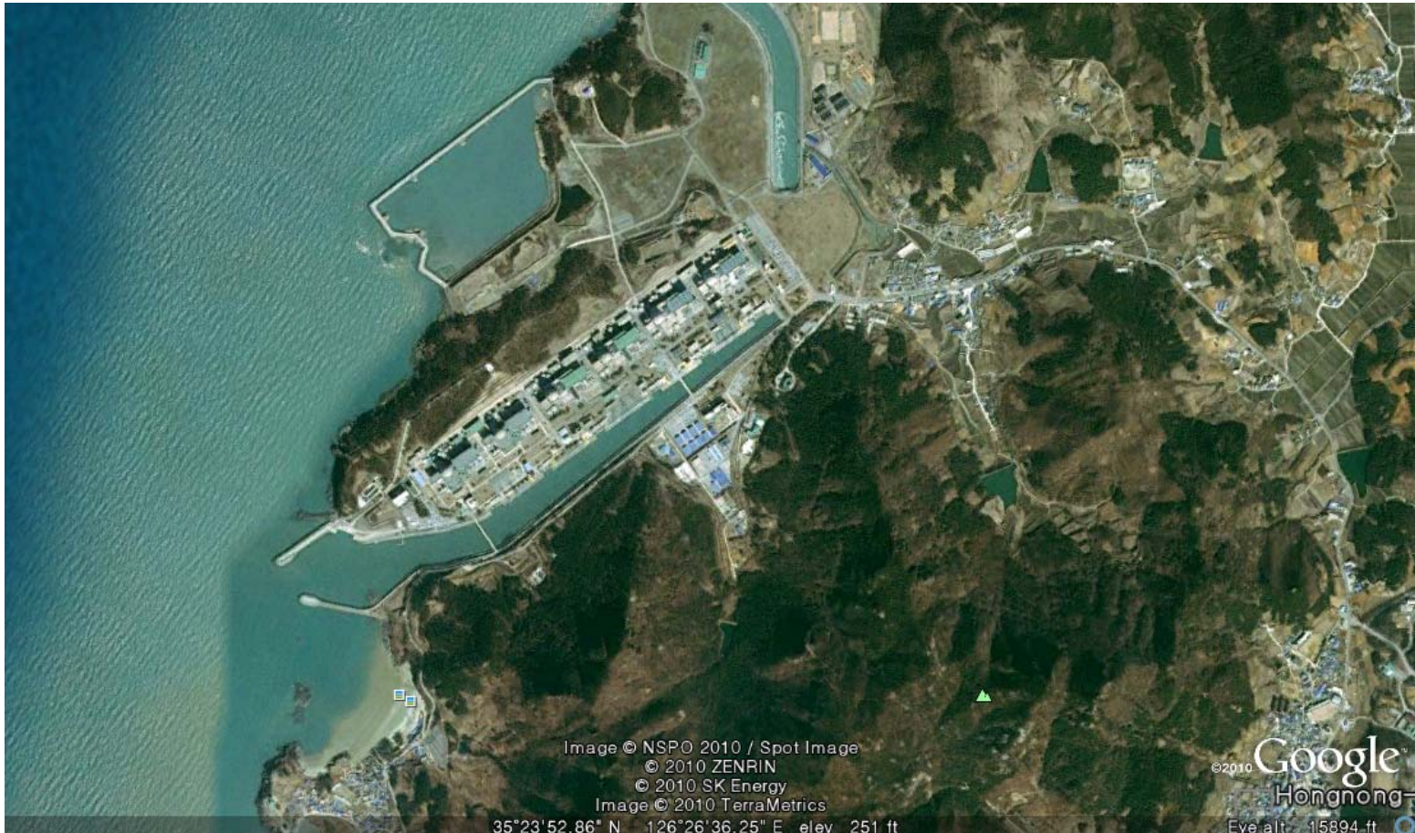
Figure. The Yonggwang nuclear power plants site (Google Earth, October 10, 2010)
