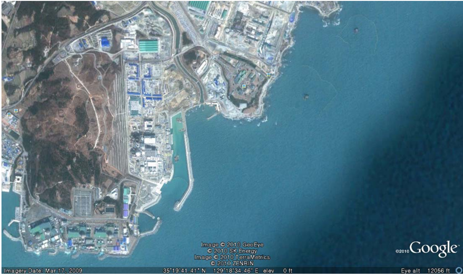
Figure. The Kori nuclear power plants site (Google Earth, October 10, 2010)
