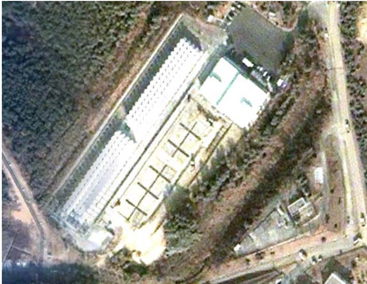
Figure. Concrete silo and MACSTOR/KN-400 at Wolsong (Google Earth, October 10, 2010)
