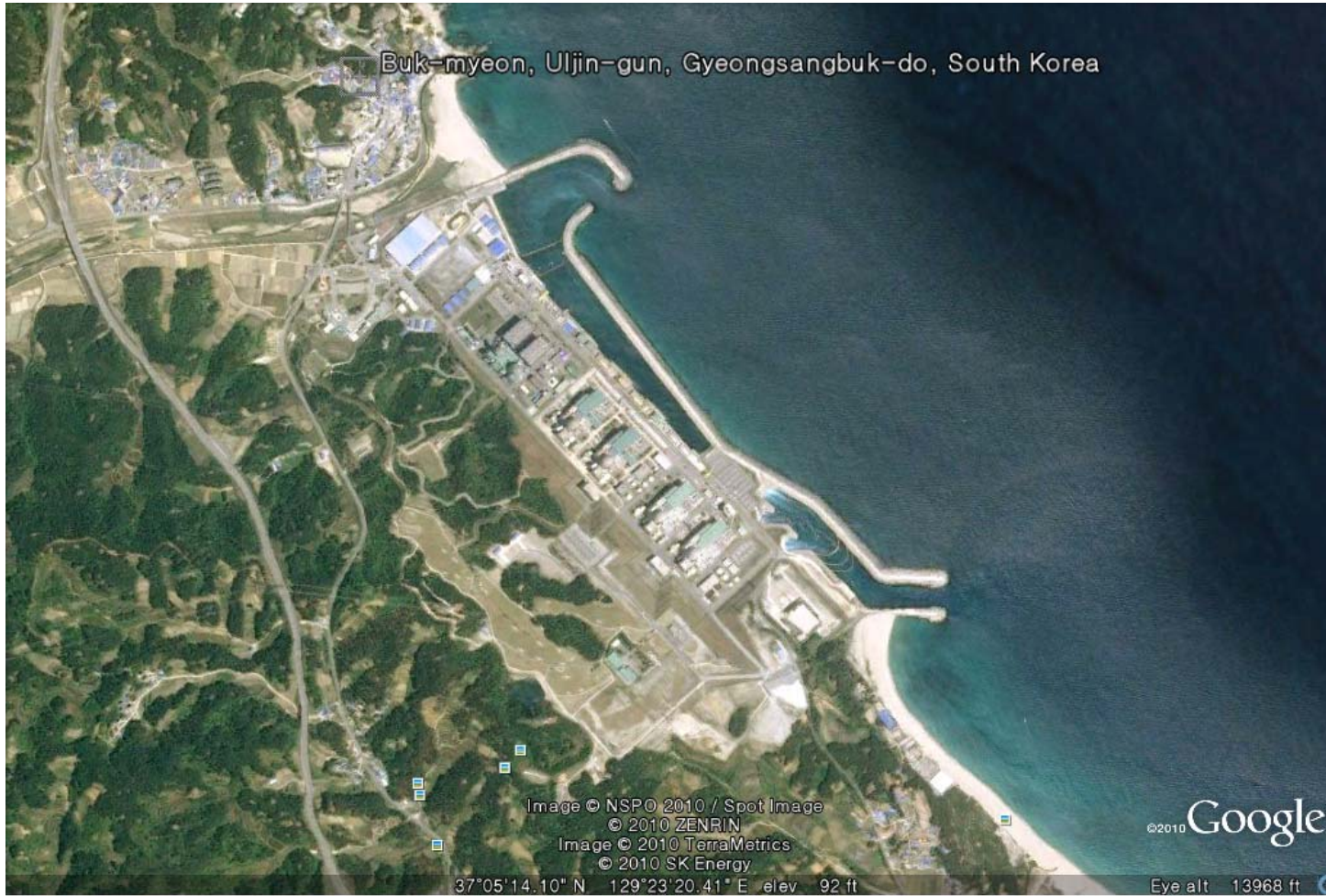
Figure. The Ulchin nuclear power plants site (Google Earth, October 10, 2010)
