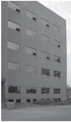
KUT Library Construction, 2004
