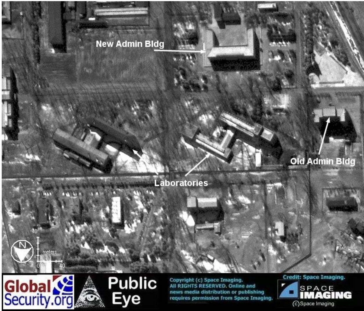
Close-up of “Support Facilities” area
